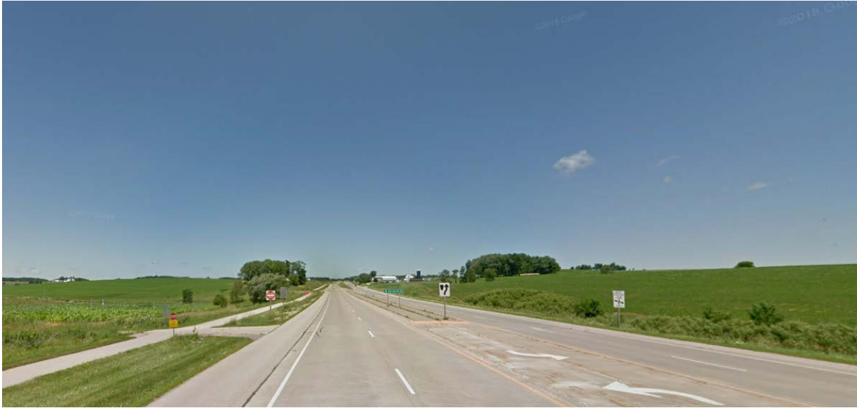
Looking north on USH 14. Cross section change from 4 lane divided highway to 5 lane undivided highway. Located approximately 550 FT south of USH 14 intersection with Springville Road.
