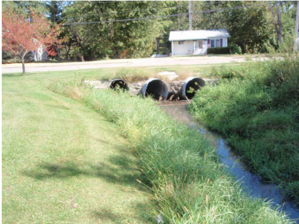
Figure 1.1 Upstream view of existing STH 89 crossing at 2 nd Ward Creek
