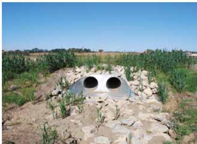
Multiple-Inlet End Sections greatly improve appearance of culverts for an aesthetic, finished look.
