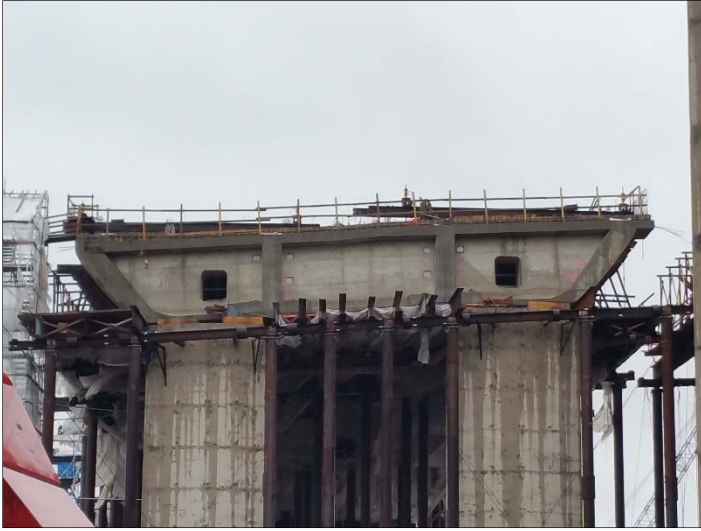
a. WB gore area: pour-backs complete, falsework removal ongoing
