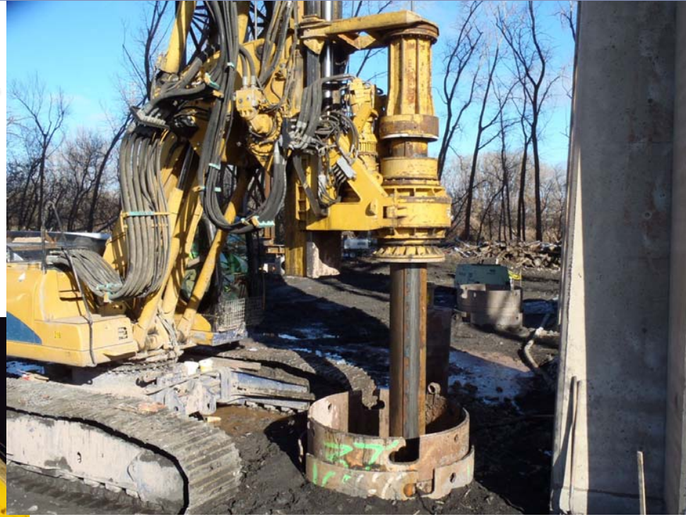
Rock Auger at Pier 22 →
