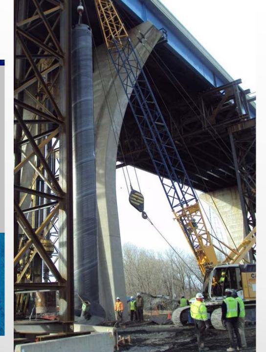
Day 68: Case installing 30-foot fiberglass liner AF 230
