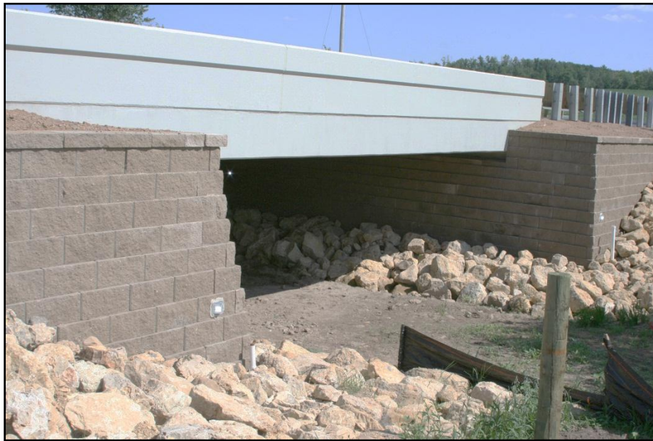
Figure 7.1-4 GRS-IBS Structure
