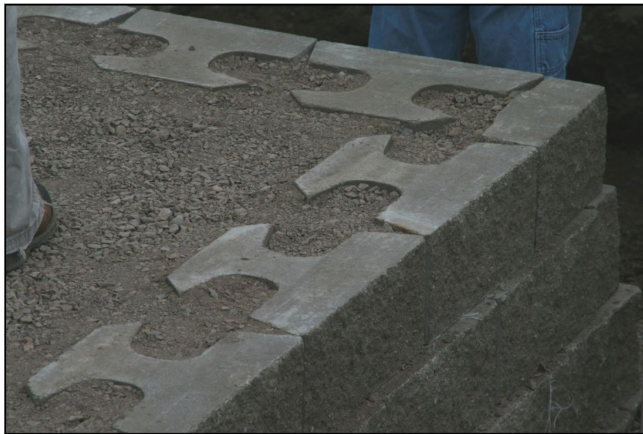
Figure 7.1-5 GRS Abutment Layer During Construction
