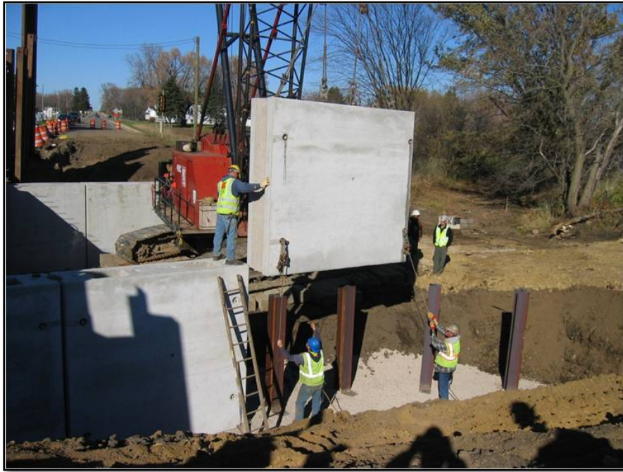
Figure 7.1-2 Prefabricated Abutment
