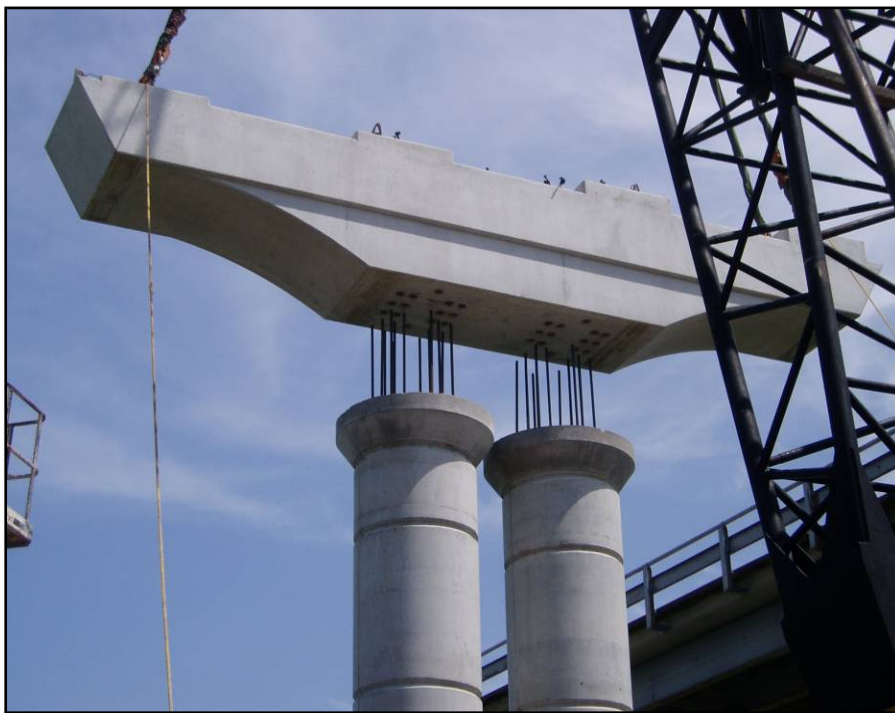
Figure 7.1-1 Prefabricated Pier Cap
