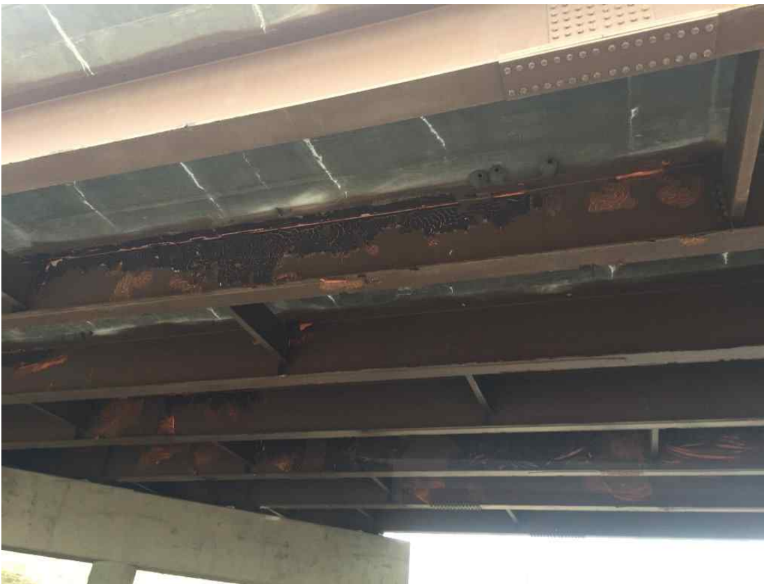
Underside of deck showing cracks with efflorescence.
