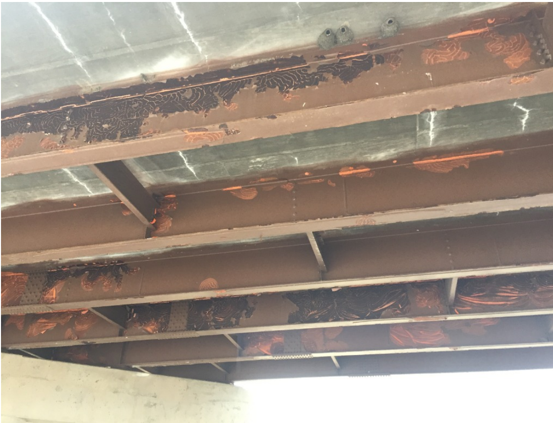
Underside of deck showing cracks with efflorescence.
