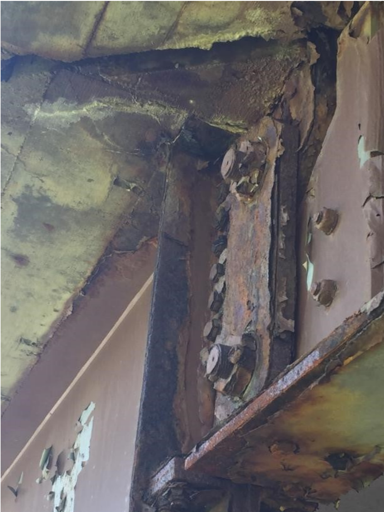
Girder 1 – pin and hanger corrosion
