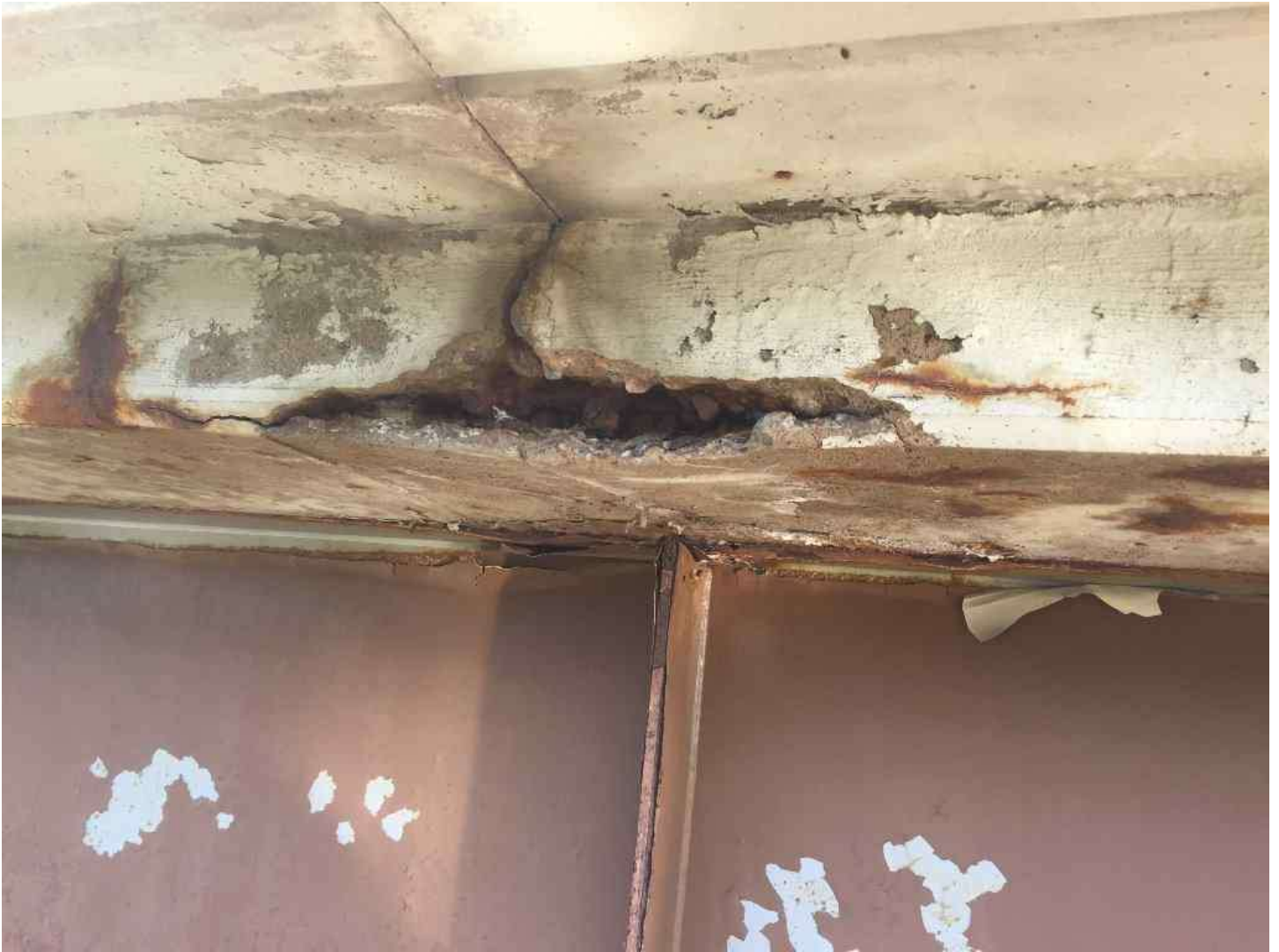
West edge of deck - spalling
