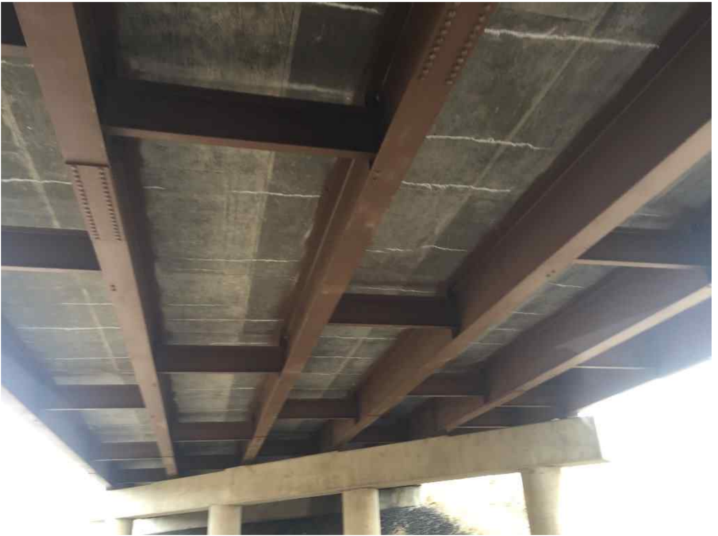
Underside of deck showing cracks with efflorescence.
