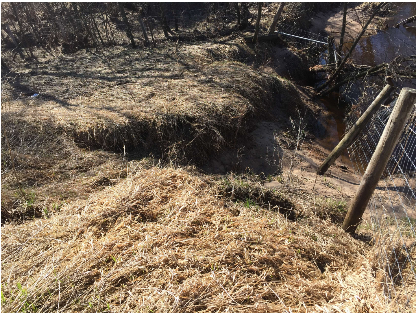
SE Corner of Structure – Streambank Erosion
