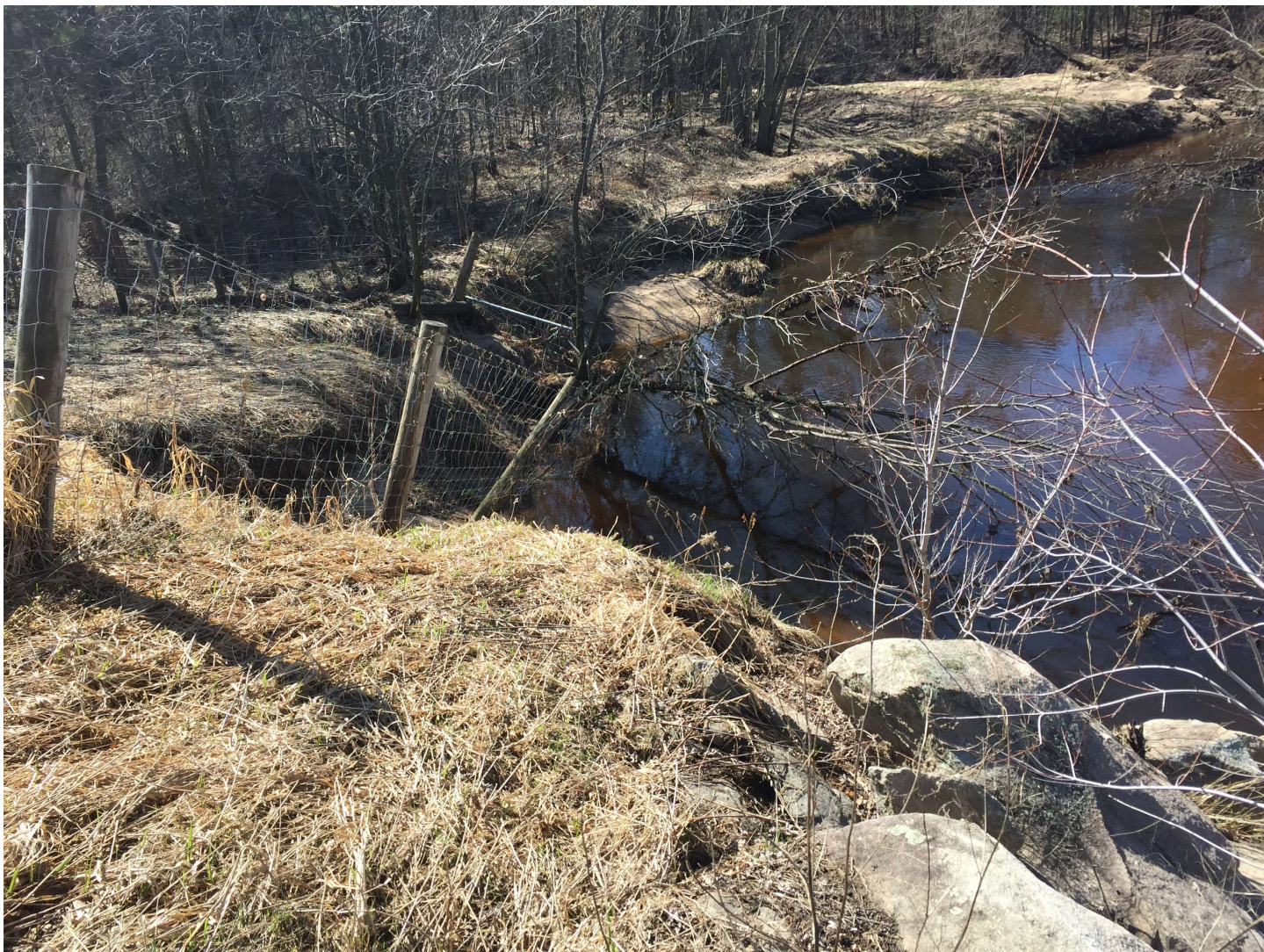
SE Corner of Structure – Streambank Erosion
