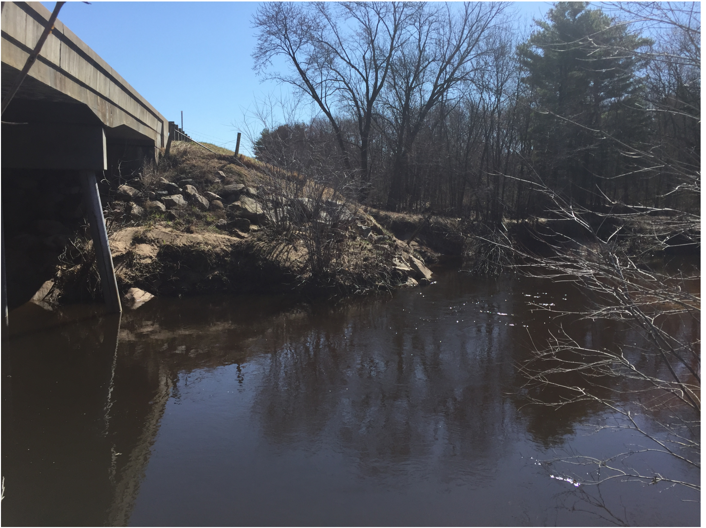
SE Corner of Structure – Streambank Erosion
