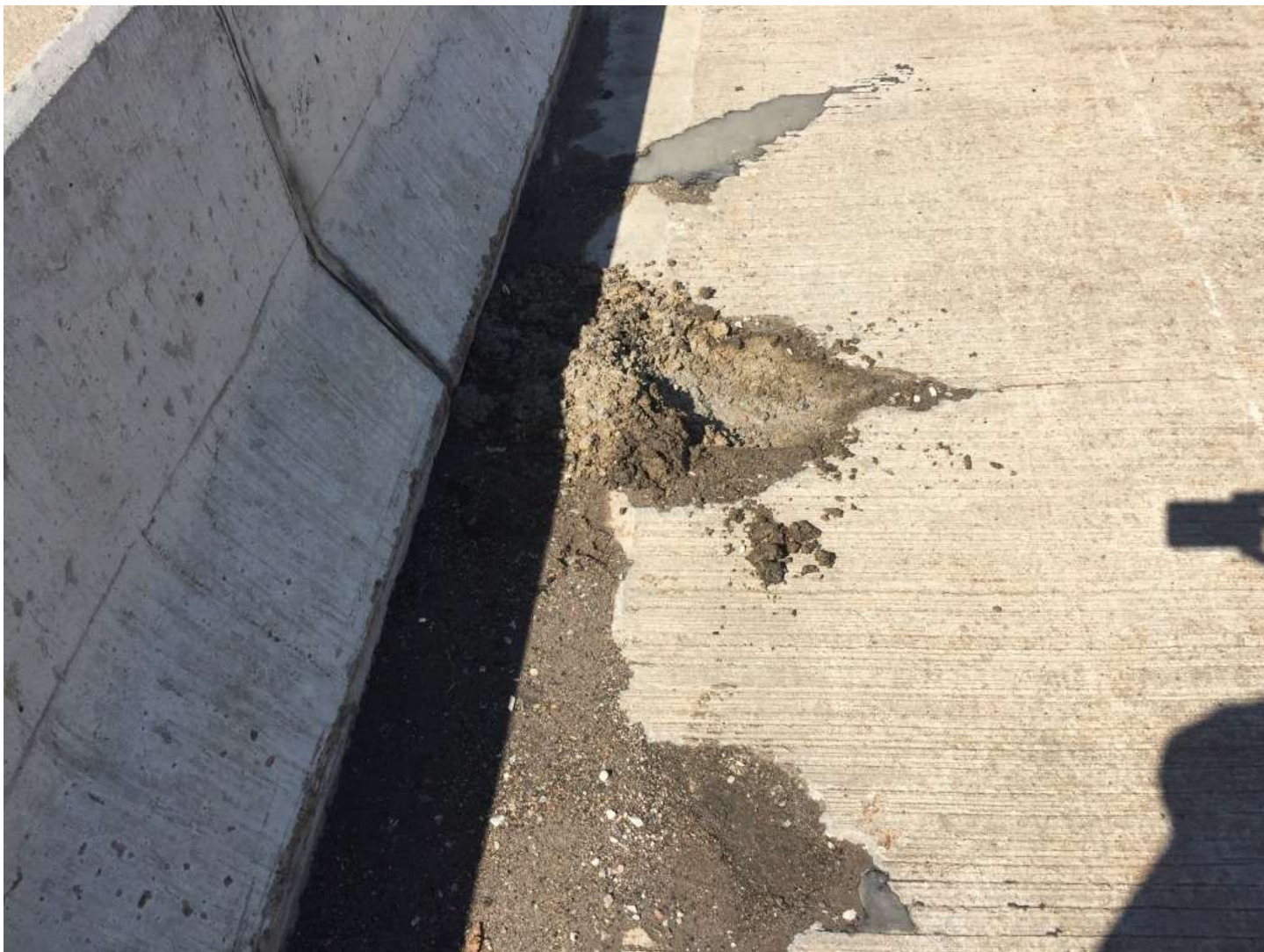
Top of deck near south rail over pier 2 - Spalling
