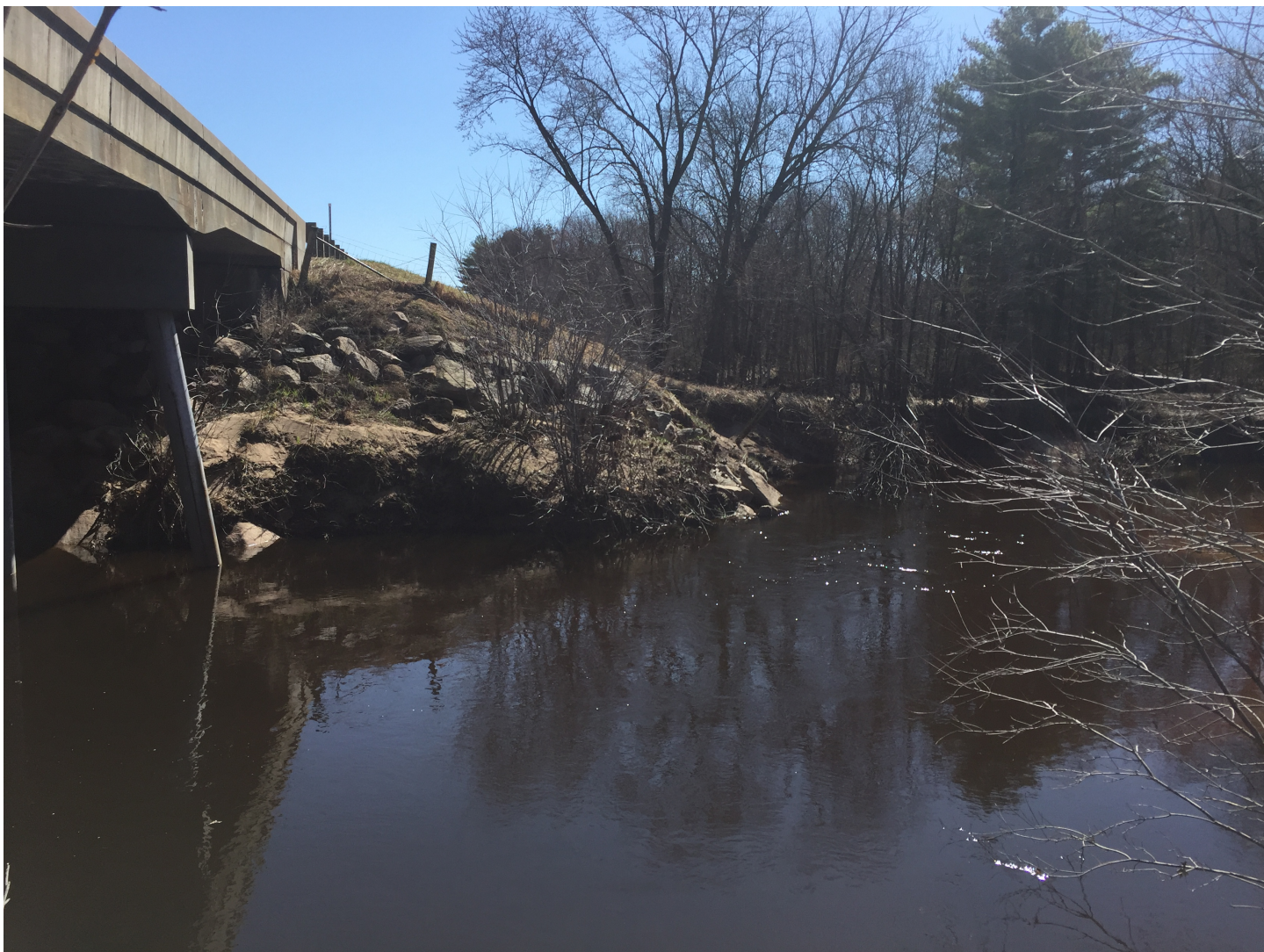
SE Corner of Structure – Streambank Erosion
