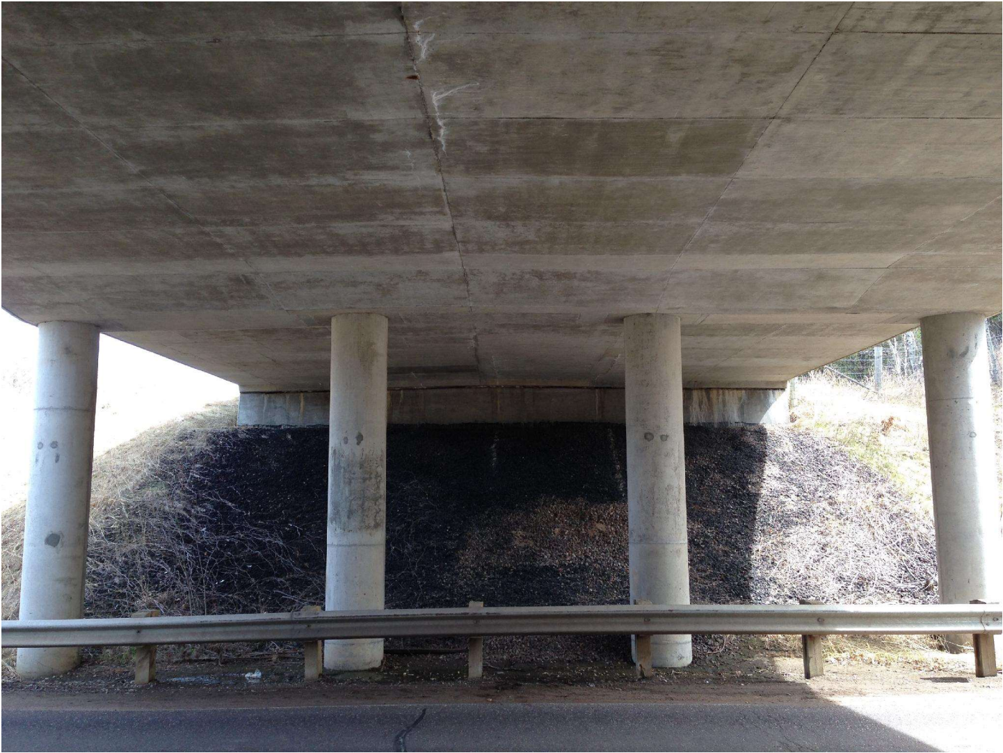
Underside of center span - Cracking
