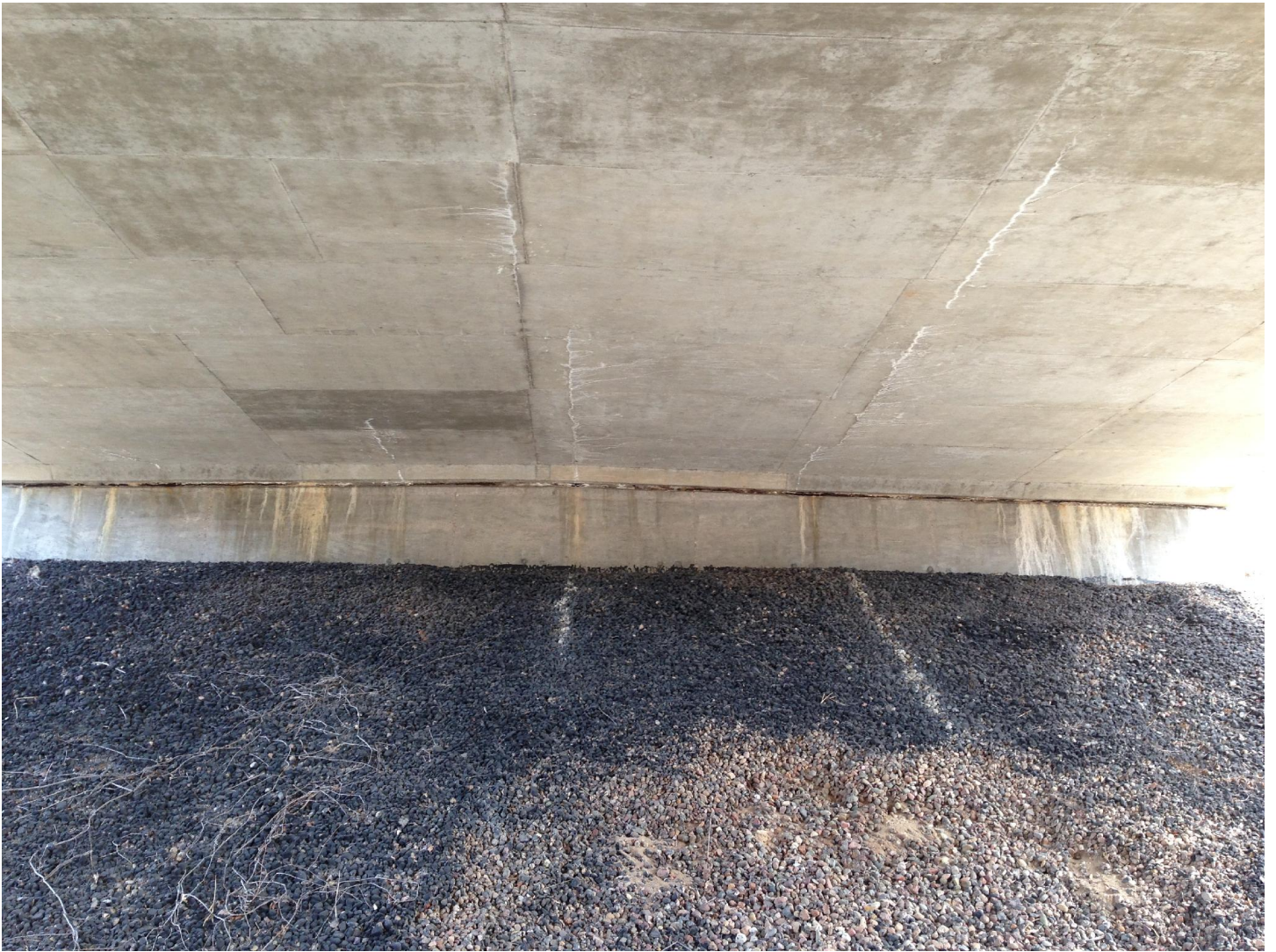
Underside of east span - Cracking
