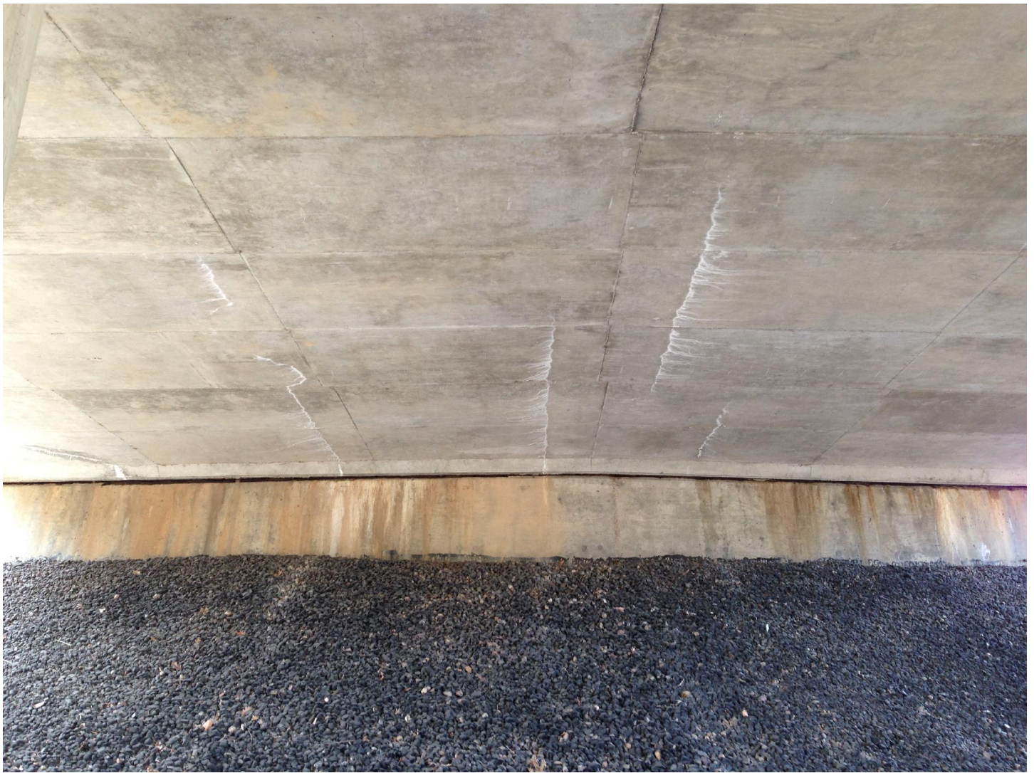
Underside of west span - Cracking
