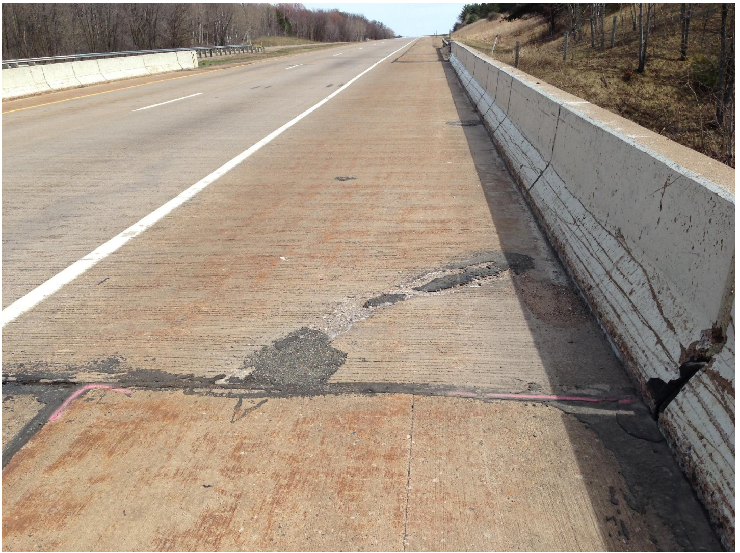
SW end of deck – Spalling and patch on edge
