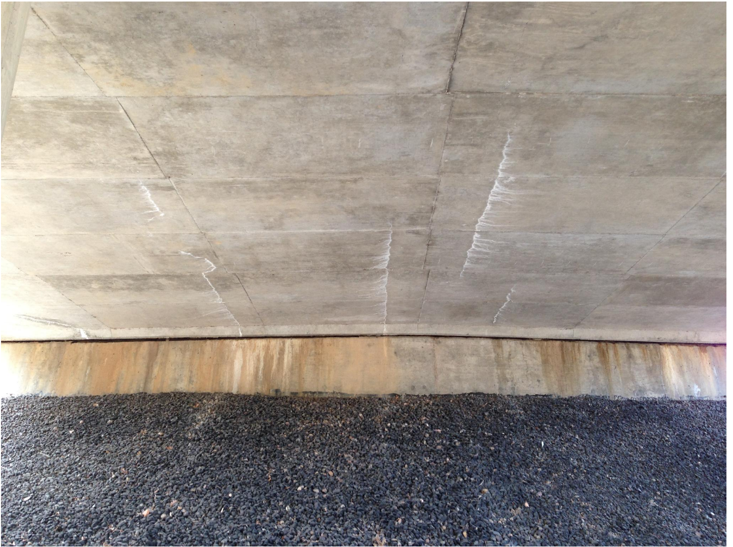
Underside of west span - Cracking
