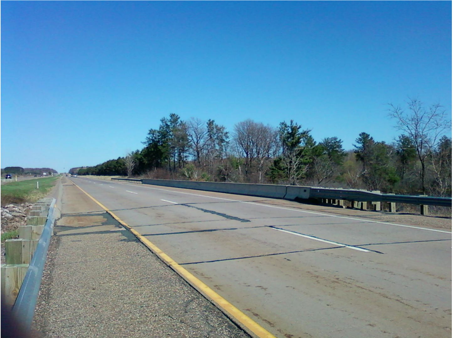
Top of Deck – Delamination and Cracking
