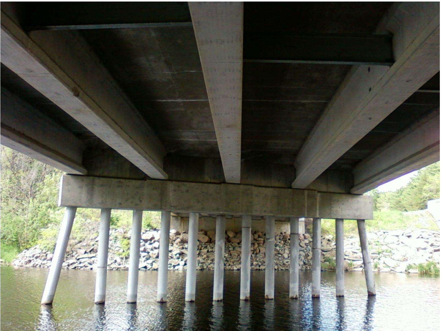
Underside of Deck – Transverse Cracks with Efflorescence
