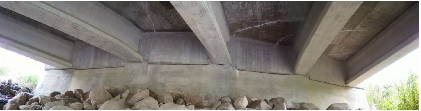
Underside of Deck – Diagonal Cracks with Efflorescence
