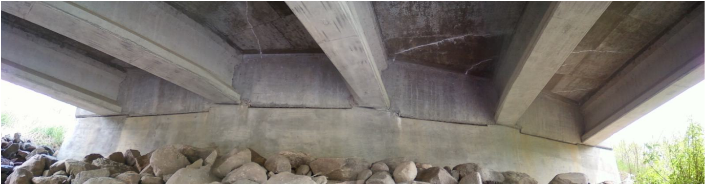
Underside of Deck – Diagonal Cracks with Efflorescence
