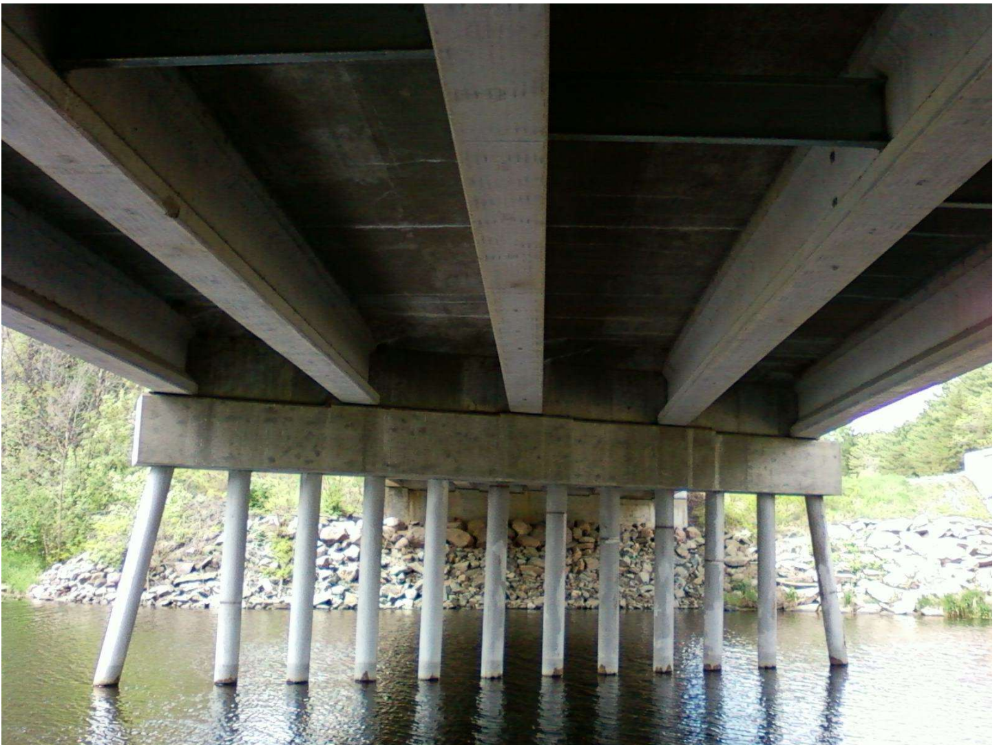
Underside of Deck – Transverse Cracks with Efflorescence
