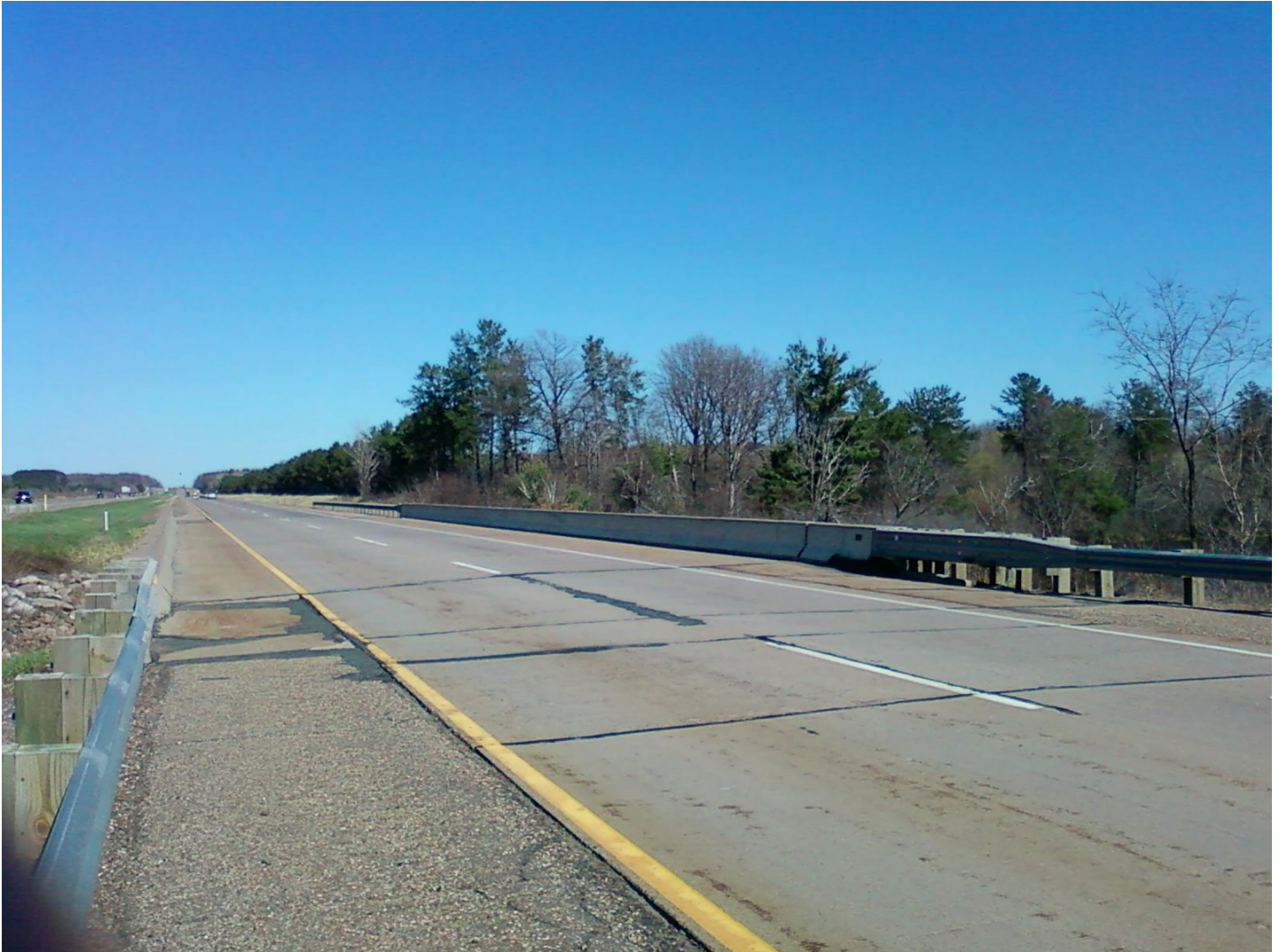
Top of Deck – Delamination and Cracking
