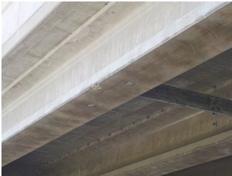
Bridge B-67-325 Exterior Girder Bottom Flange Damage
