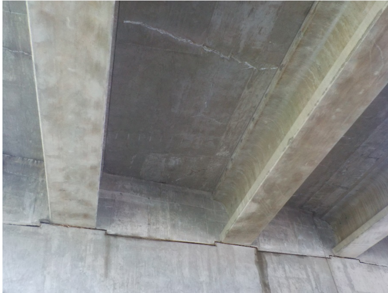
Bridge B-67-325 East Abutment Diaphragm & Bottom of Deck Cracks
