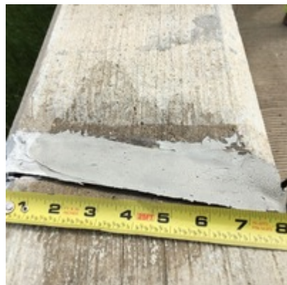
Caulk in abutment joint
