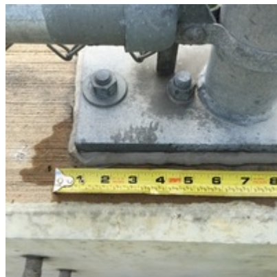
Caulk around pedestrian fence attachment plates on parapet (did not observe any gaskets under plate)
