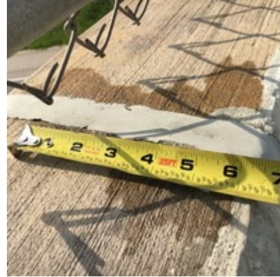
Caulk in parapet expansion joint
