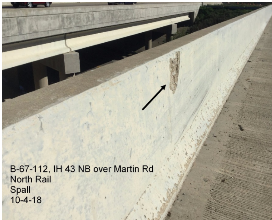
North Rail, Spalls. Photo from WisDOT inspection report.
