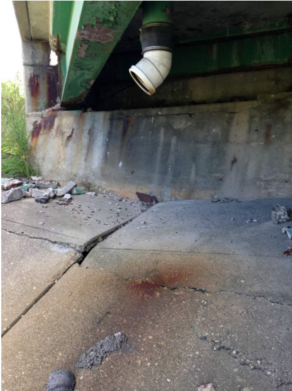
South abutment and heaved slope paving. Note daylight shining through gap in backwall.
