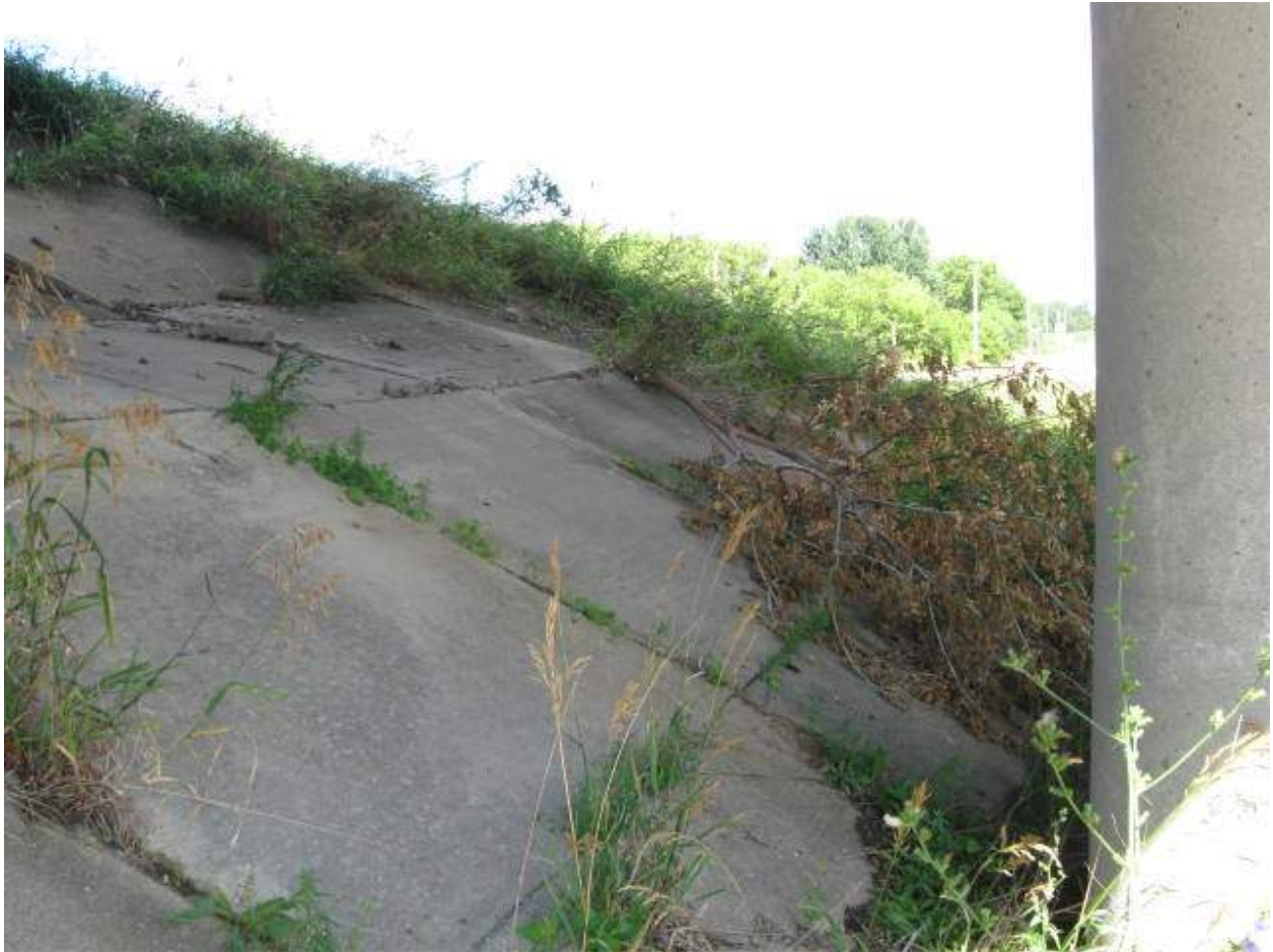
North slope paving, cracked and heaved
