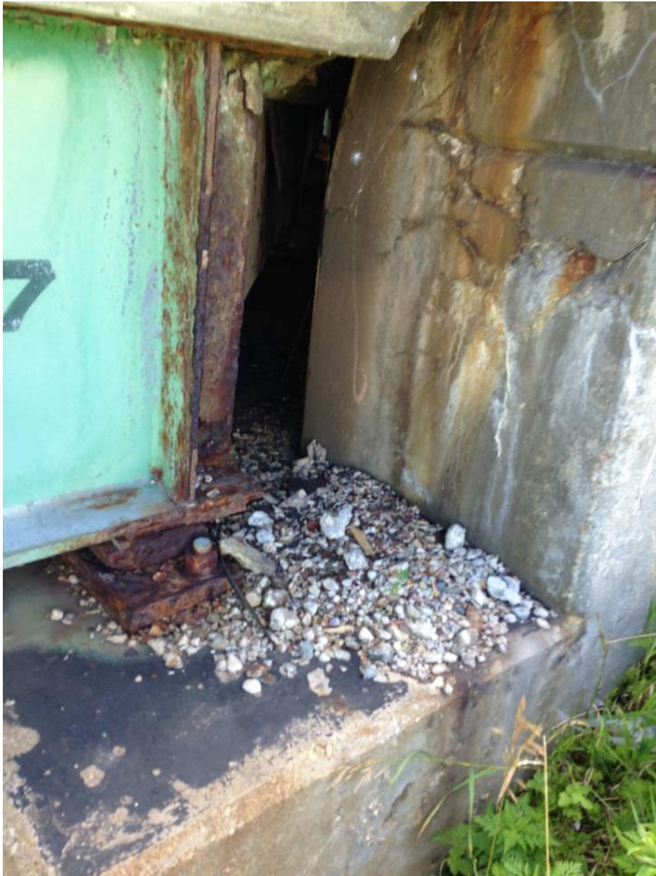
North abutment, east end. Deteriorated backwall, girder and, and bearing.
