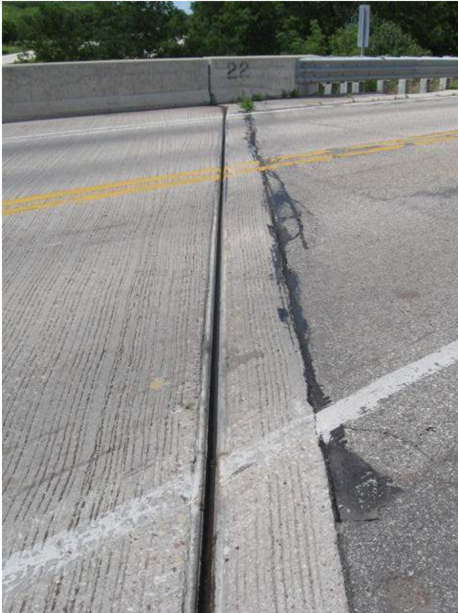
North expansion joint, looking east. Portions of paving block higher than deck.
