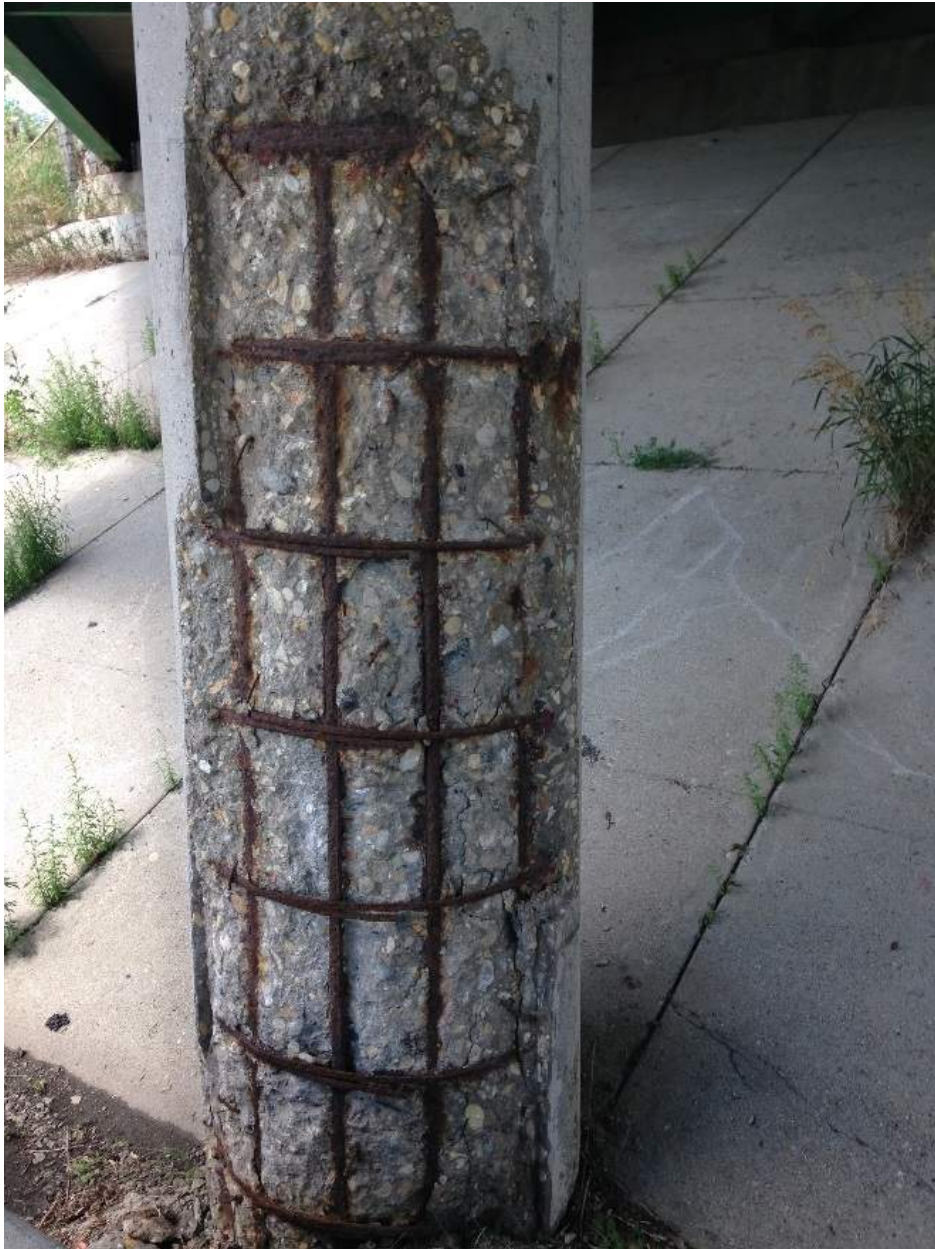
Exposed rebar at failed column repair. Typical several columns at the shoulder piers.
