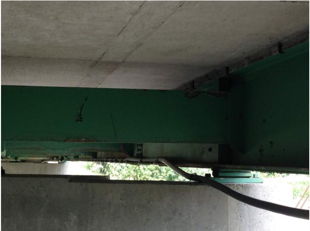
Utility (abandoned?) attached to east girder
