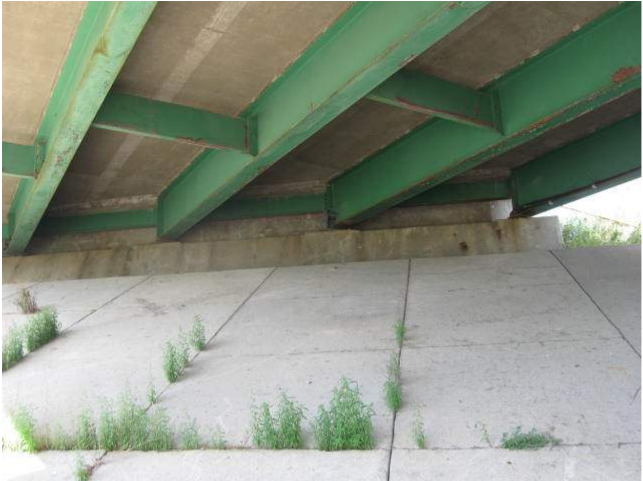
North abutment and slope paving
