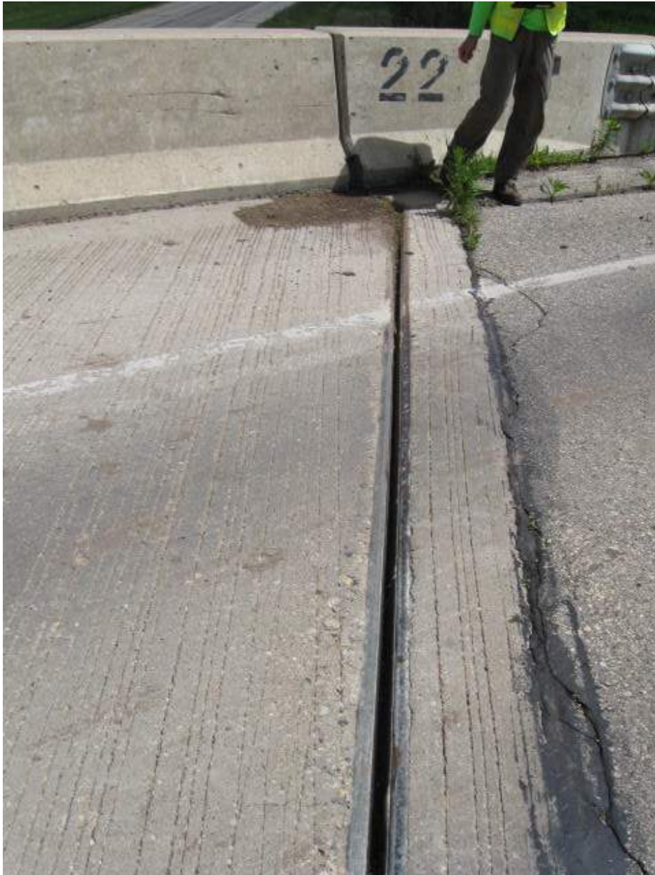
South expansion joint, looking east. Paving block higher than deck slab. Evidence of drainage issues.
