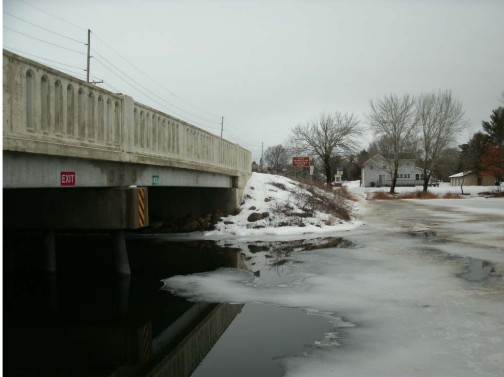
Figure 20: Northeast corner of bridge rip rap
