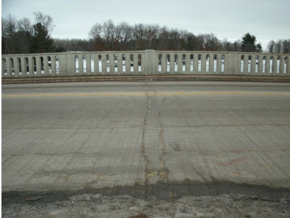
Figure 10: Center of bridge structure crack line looking East
