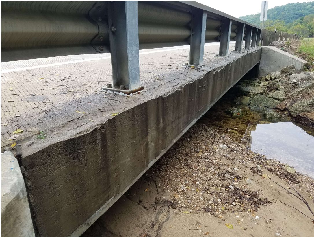
Spalling Concrete along north edge of deck
