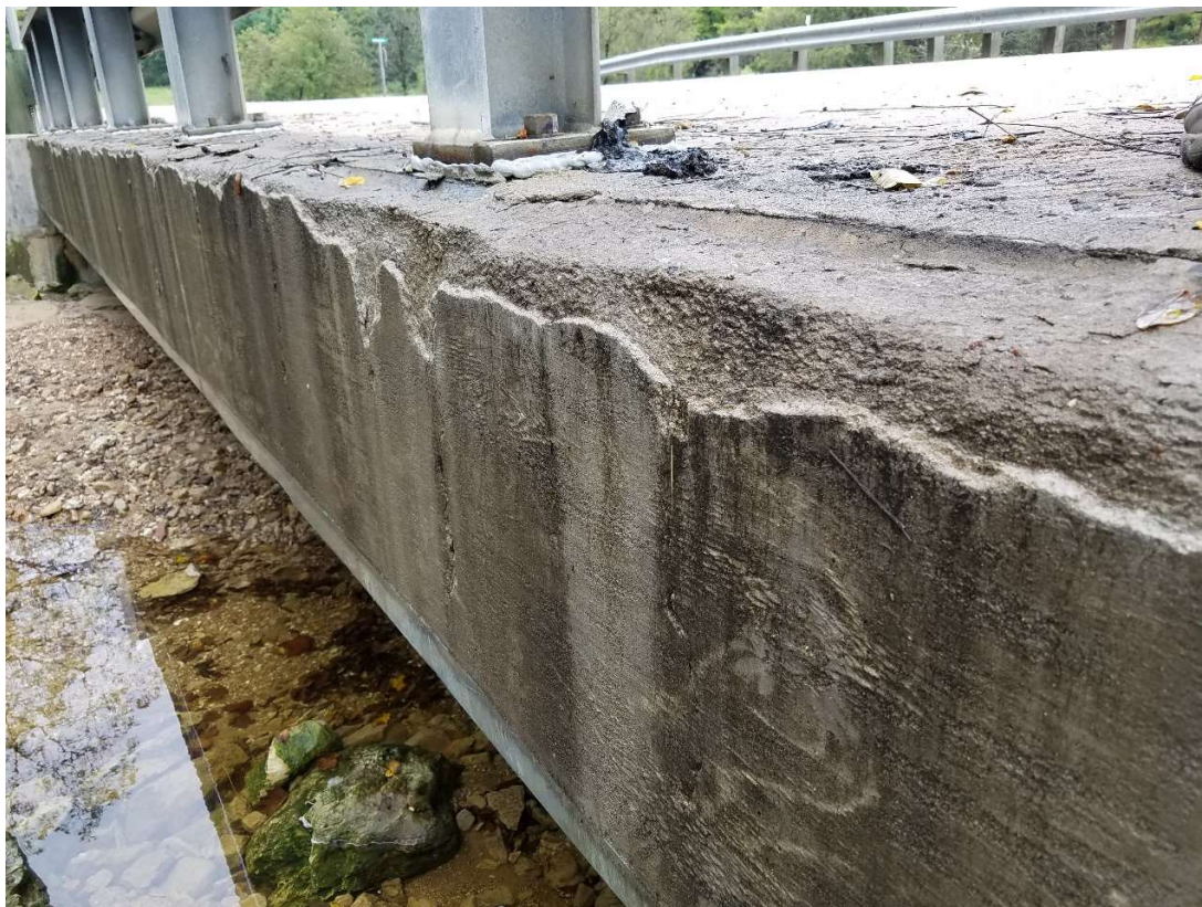
Spalling Concrete along north edge of deck
