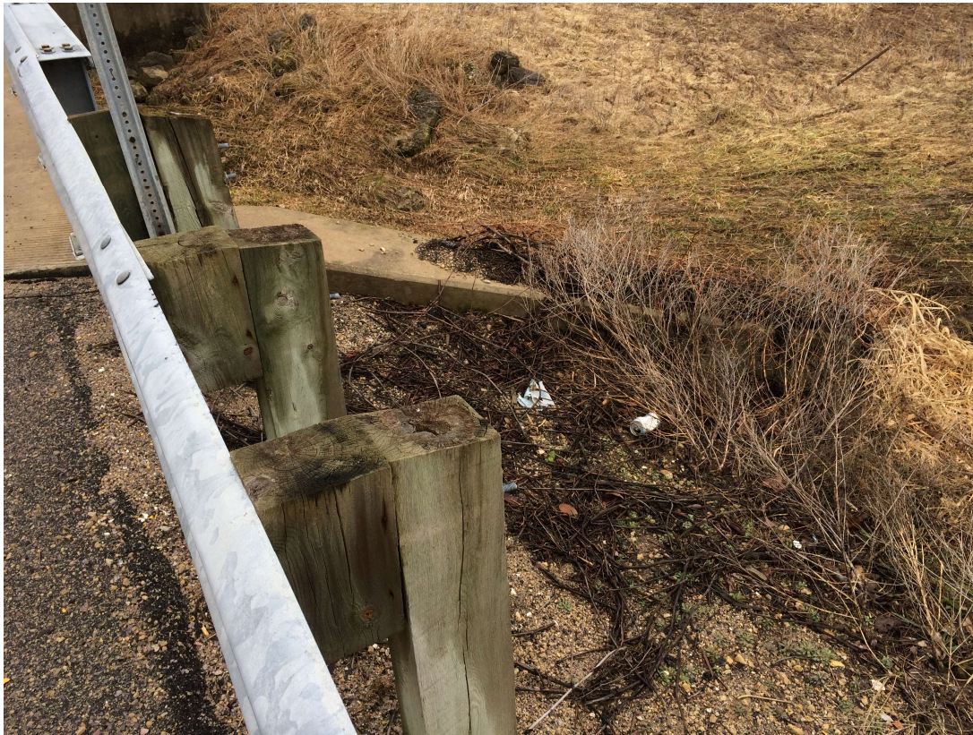
Rotten guardrail posts on bridge approach
