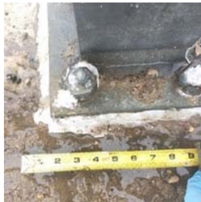
Caulk around railing attachment plate
