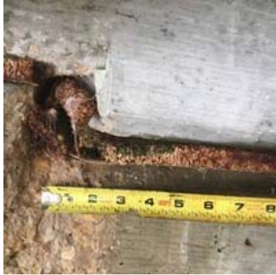
Cork-like material in abutment joint
