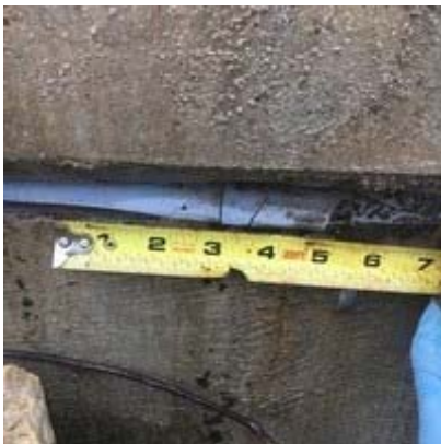
Plastic-like material in abutment joint
