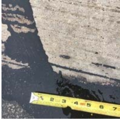
Tar-like material in bridge deck expansion joint
