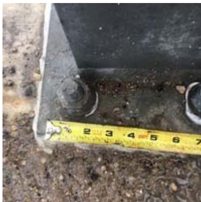
Caulk around nuts and bolts in railing attachment plate
