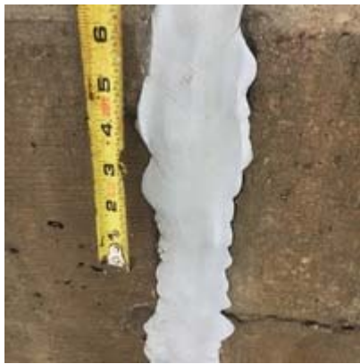
Caulk in abutment joint
