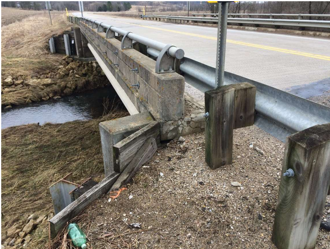
NW Corner - Guardrail to Parapet Connection, Deteriorated curb (Looking East)
