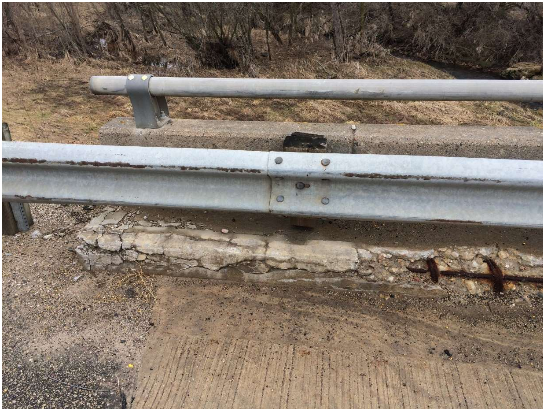
Spalling/Cracking in North Curb
