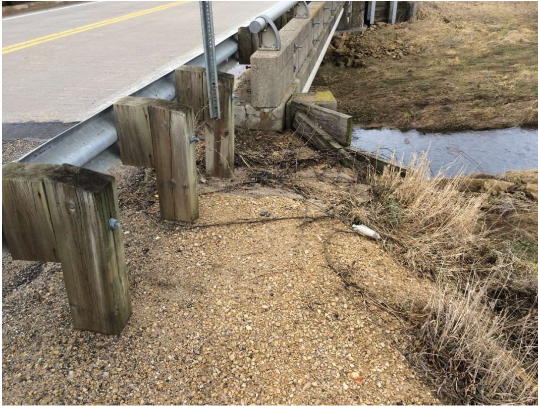
Wing 3 (NE Wing), Shoulder Erosion (Looking West)
