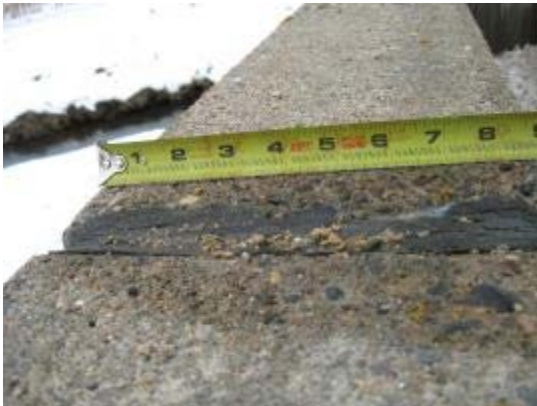
Caulk in parapet expansion joint
