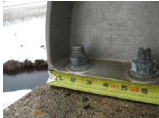
Caulk around bolts in attachment plate
