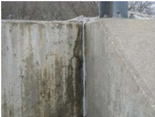
Caulk in wingwall joint
