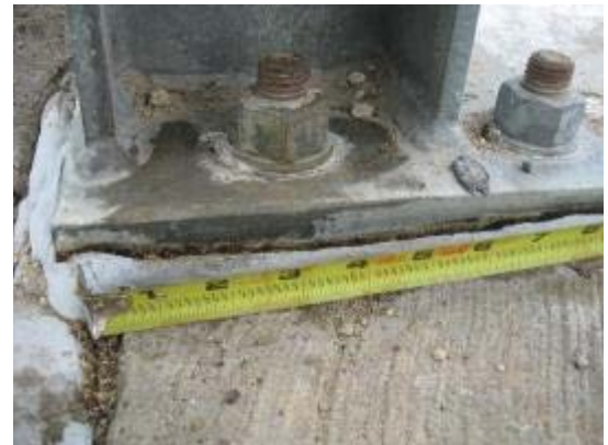
Caulk around railing attachment plate and around bolts in plate
