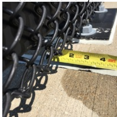
Caulk in parapet joint
