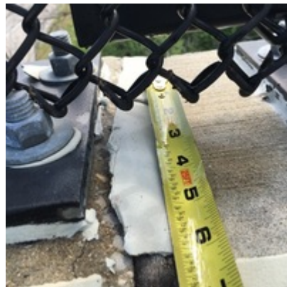
Caulk in abutment joint
