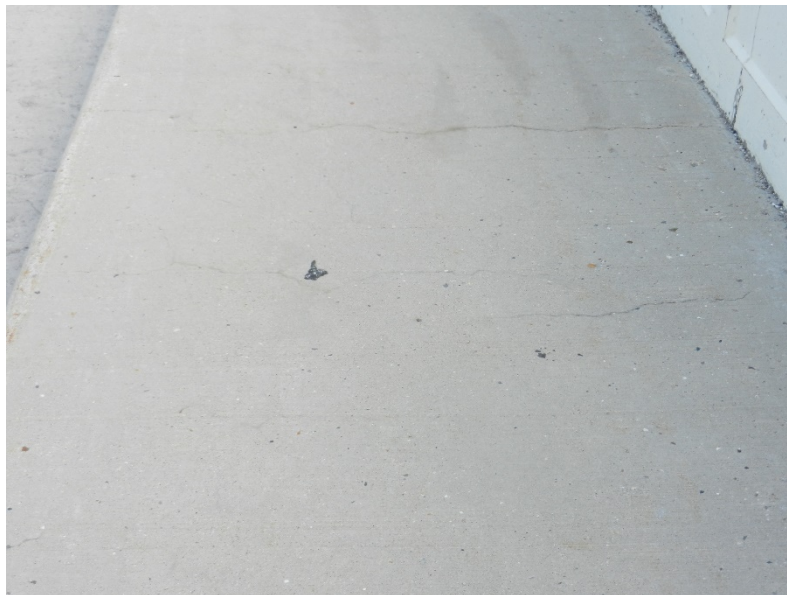
Bridge B-40-376 Sidewalk Cracks
