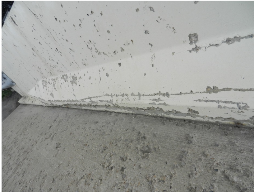
Bridge B-40-376 SW Corner Parapet Scaling & Cracking
