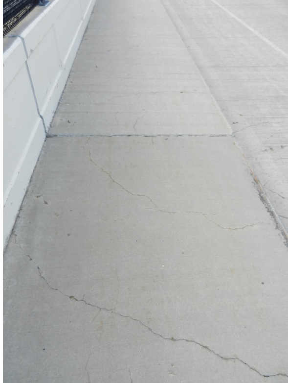
Bridge B-40-376 Sidewalk Cracks
