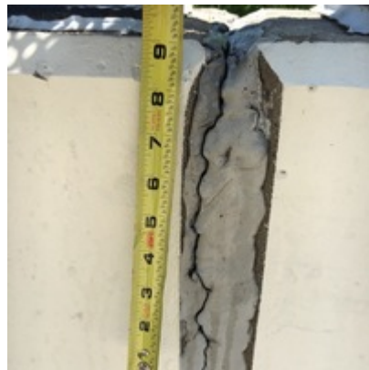
Caulk in abutment joint
