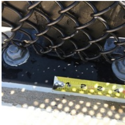
Caulk around pedestrian fence attachment plate and around bolts in plate (did not observe any gaskets under plate)
