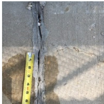
Caulk in parapet and sidewalk joints
