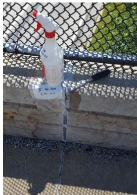
Caulk in parapet expansion joint and sidewalk joint
