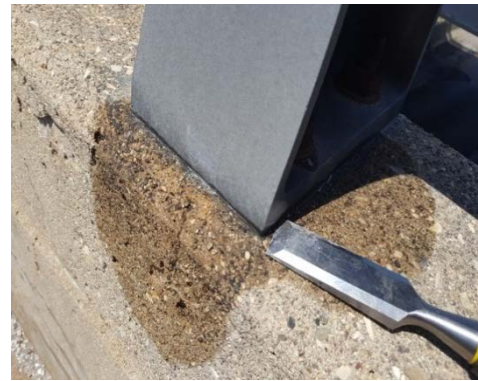
Gasket under railing attachment plate
