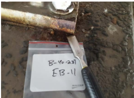
Tar on bearing support piers
