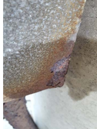
Paint on galvanized metal conduit
