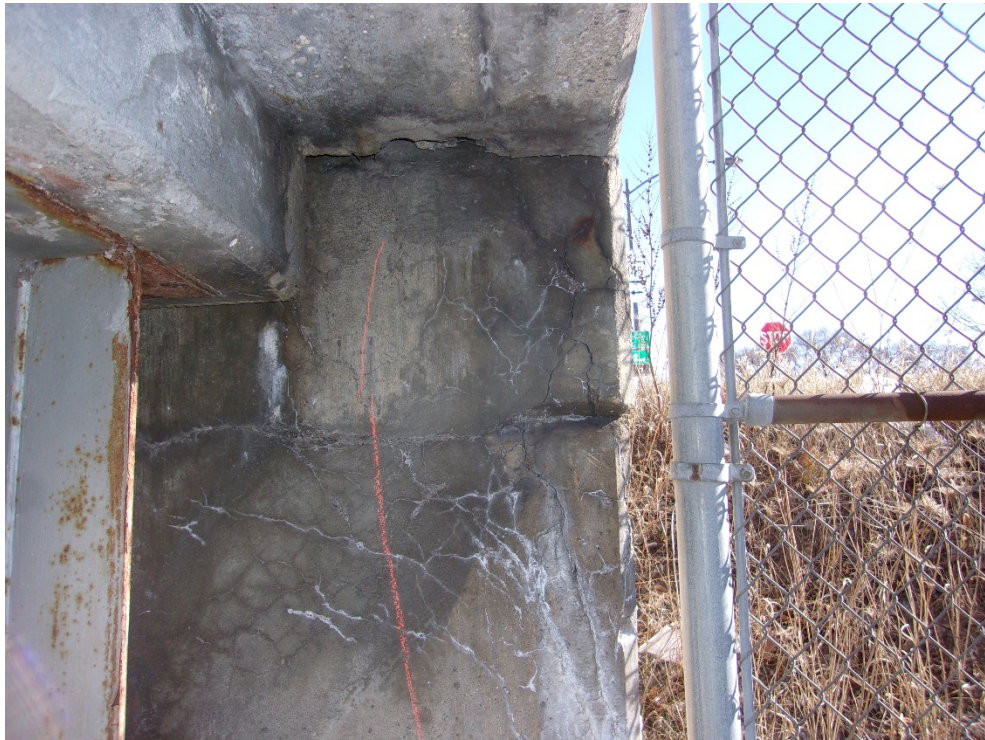
13) Leaching map cracking at southeast corner of east abutment backwall
