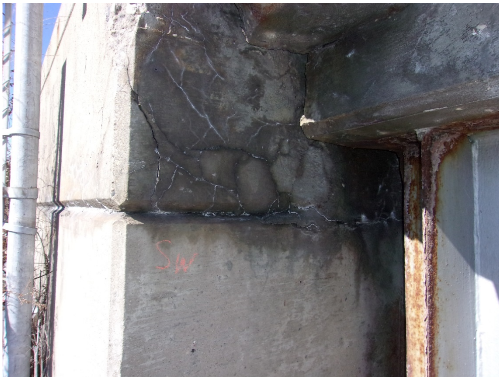
32) Leaching map cracks at southwest wingwall/abutment backwall
