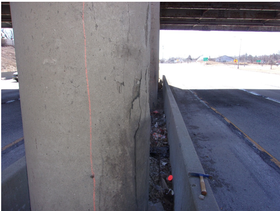
22) Large delam at Pier 3 column
