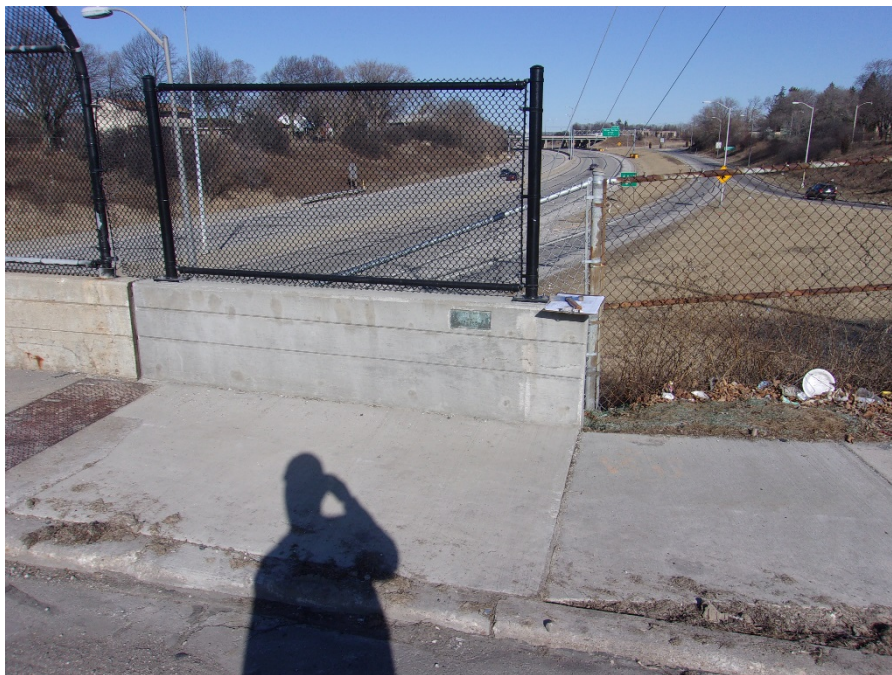
2) Inside face of northeast wingwall, replaced 09/2017, looking north
