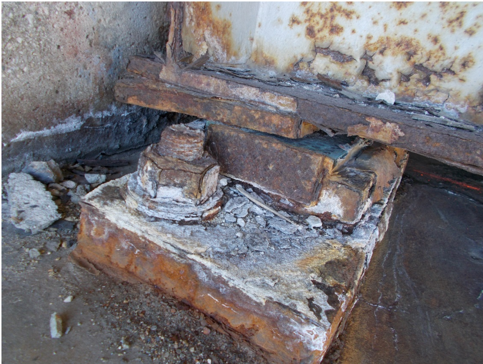
16) Girder 1 east abutment bearing condition, top plate is excessively beyond bearing anchorage. Bronze plate is exposed.
