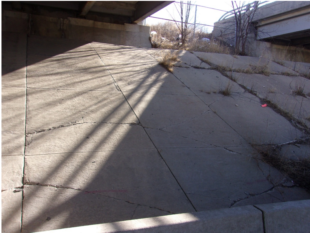
11) Slope paving condition in front of east abutment
