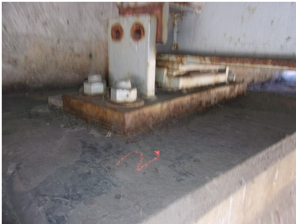
30) Girder 2 west abutment bearing condition. Missing bolts at hold down. Noticeable vertical displacement of hold down.
