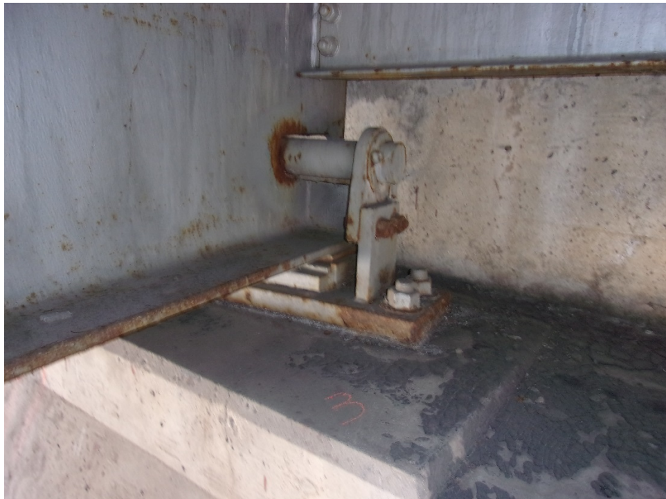
18) Girder 3 east abutment bearing condition, slot in girder is tight to hold down pin
