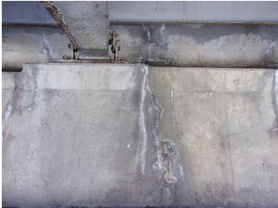
12) Typical abutment frontface/backwall deterioration at east abutment
