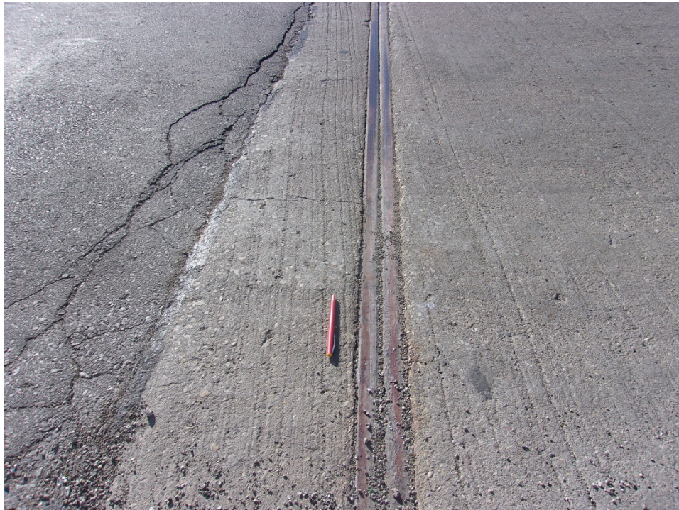
3) Expansion device at east abutment, joint is nearly closed
