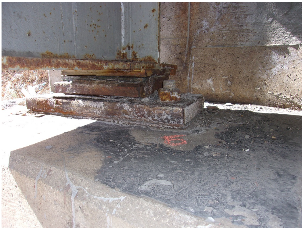
26) Girder 6 west abutment bearing condition
