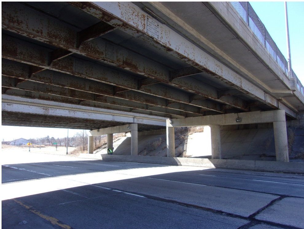
24) Girder/paint system condition state of span 2 (looking southwest)
