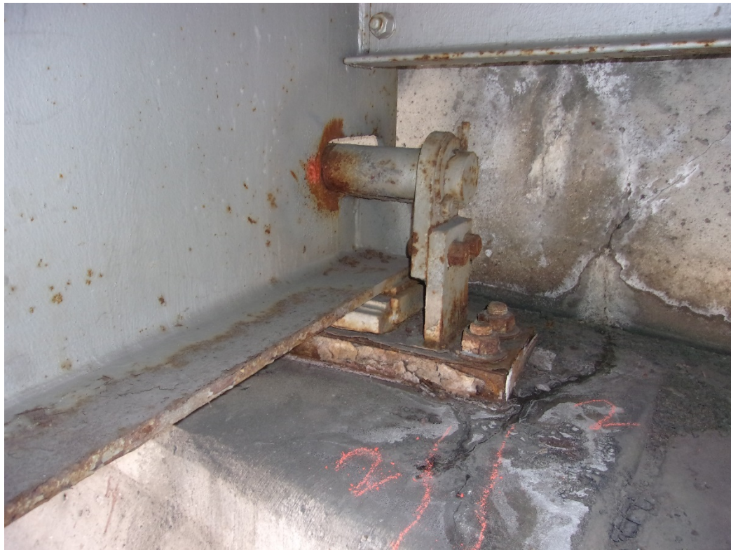
17) Girder 2 east abutment bearing condition, slot in girder is tight to hold down pin
