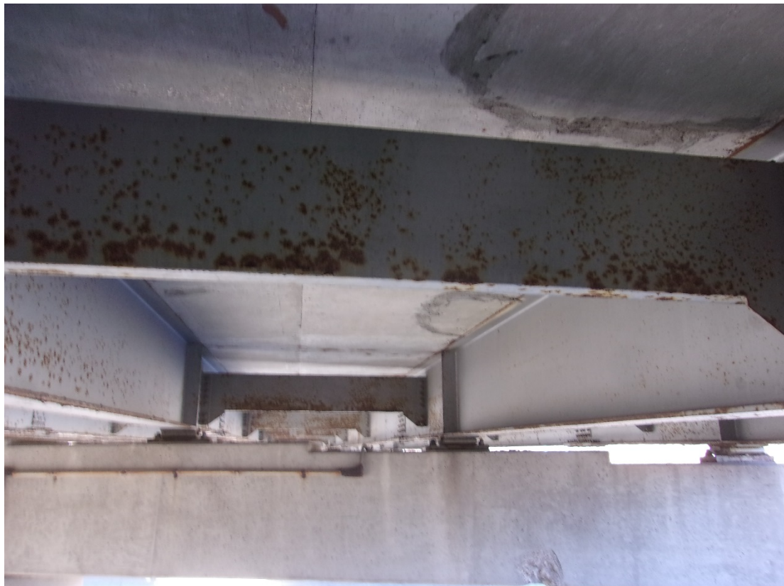
14) View of paint system condition looking west
