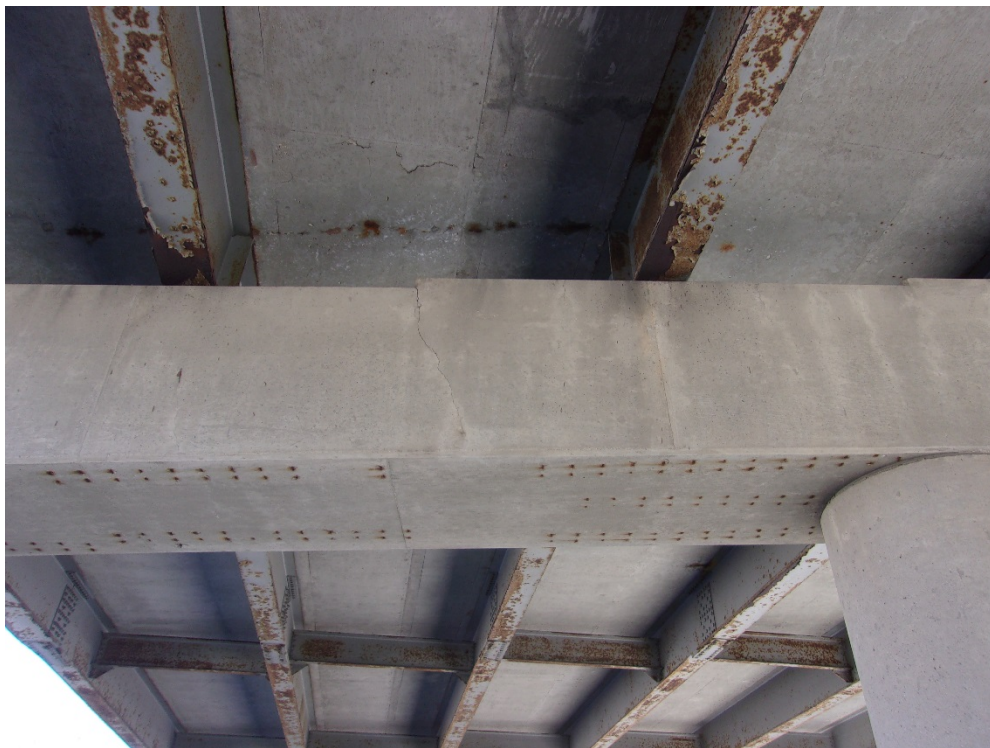
34) Vertical shear crack at Pier 2 between girders 2 and 3 (looking east)
