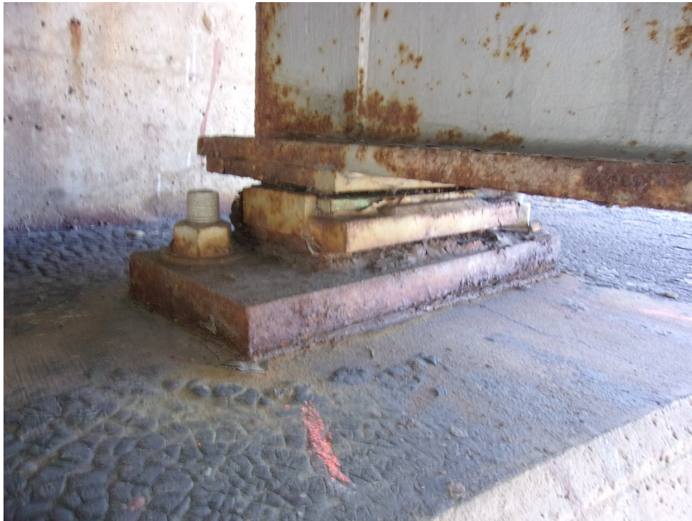
31) Girder 1 west abutment bearing condition
