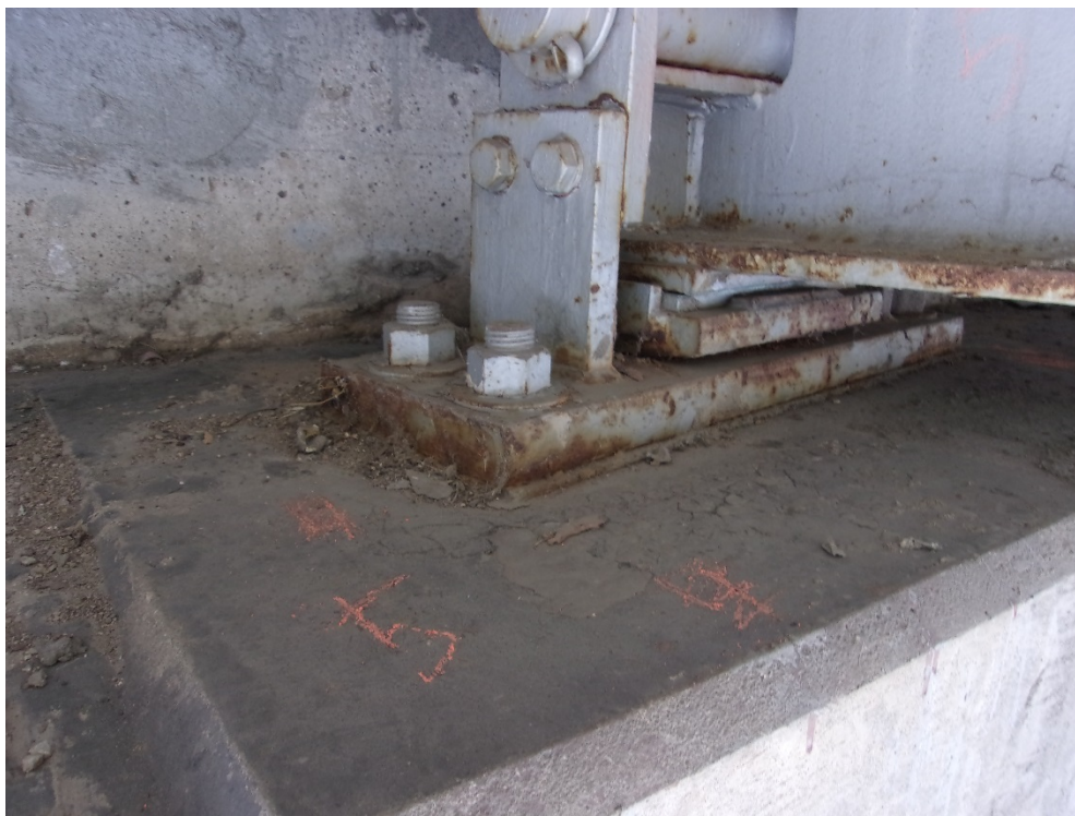
27) Girder 5 west abutment bearing condition
