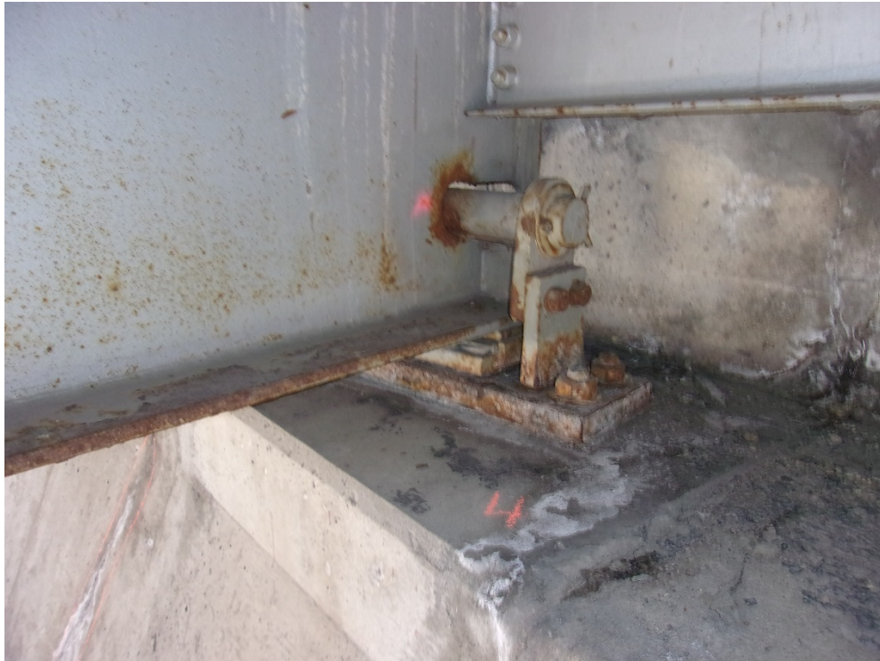
19) Girder 4 east abutment bearing condition, slot in girder is tight to hold down pin
