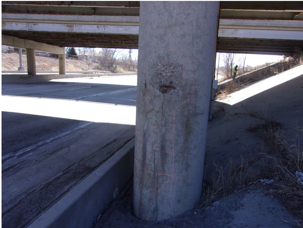
25) Delam at Pier 1 Column 1 north face
