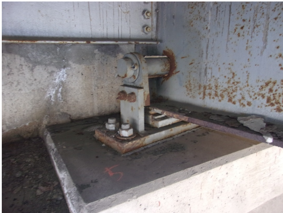
20) Girder 5 east abutment bearing condition, slot in girder is against hold down pin
