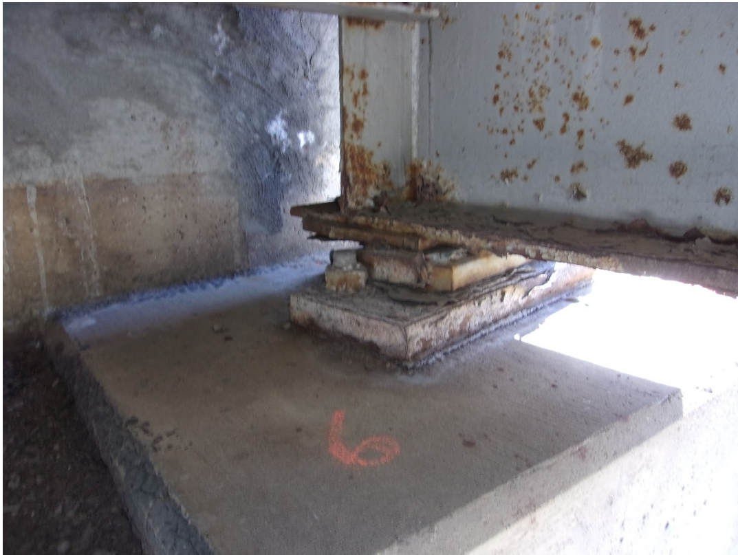
21) Girder 6 east abutment bearing condition
