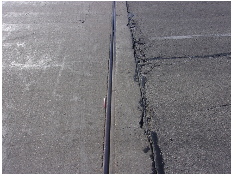
9) Expansion device at west abutment, joint is nearly closed
