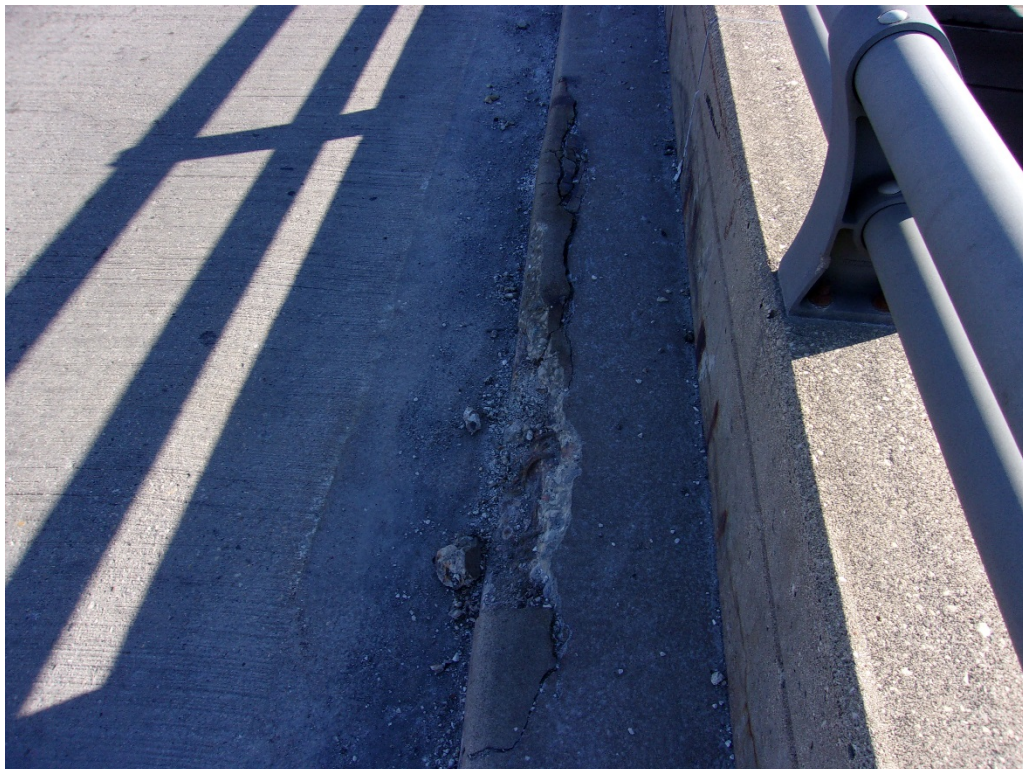
6) Curb deterioration/spall at south of structure
