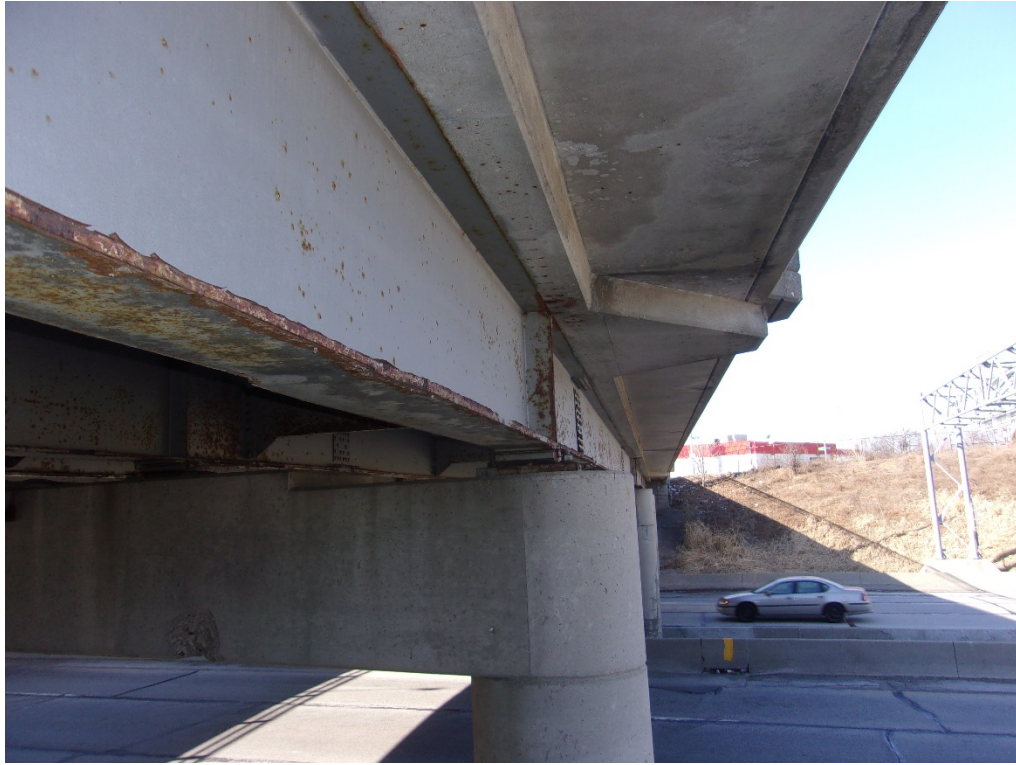
15) Fascia girder paint system condition looking west
