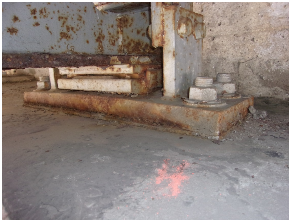
28) Girder 4 west abutment bearing condition
