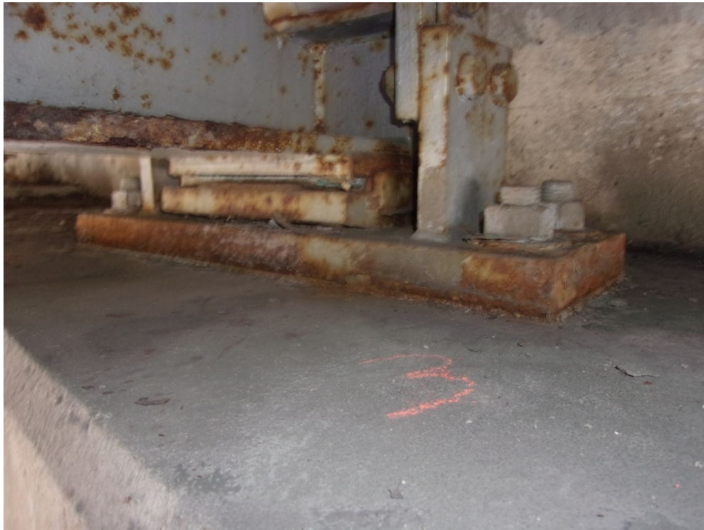
29) Girder 3 west abutment bearing condition
