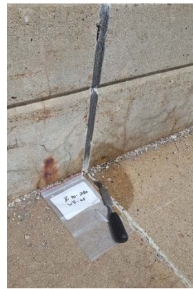
Caulk in parapet expansion joint and sidewalk joint
