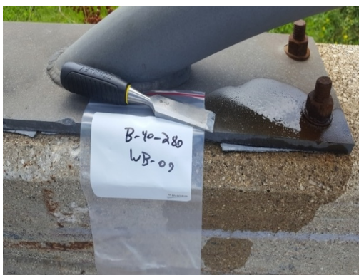
Gasket under railing attachment plate on parapet
