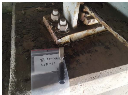
Tar on bridge bearing support piers
