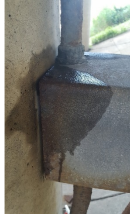
Silver paint on galvanized metal conduit
