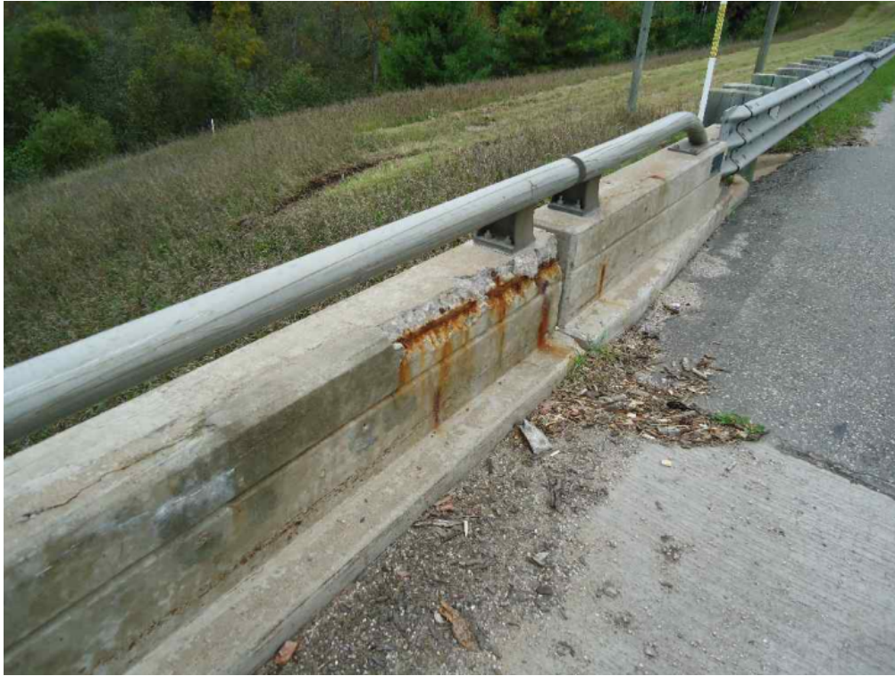
Spalling at West parapet at North end of bridge
