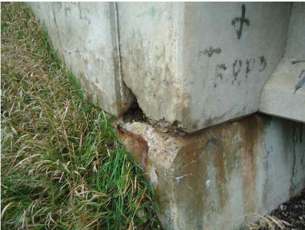
Spalling at West corner of North abutment
