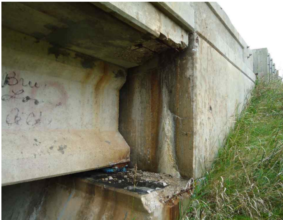
Spalling at West corner of South abutment
