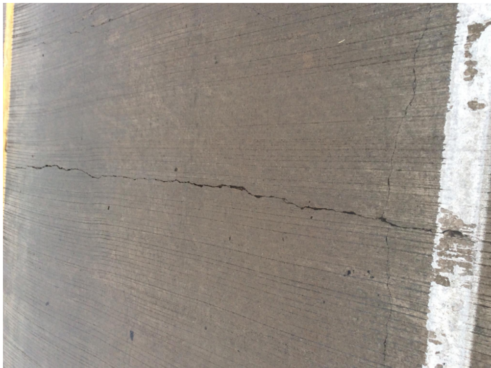
Deck cracking over piers
