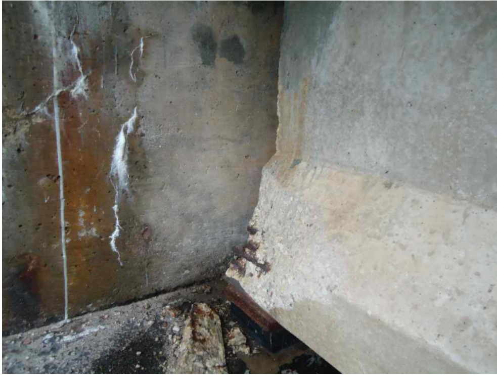
Spalling in Girder 5 at South abutment
