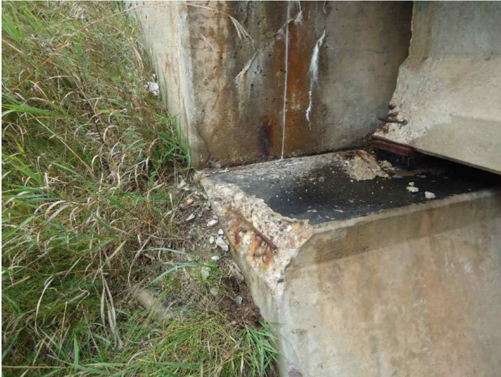
Spalling at East corner of South abutment
