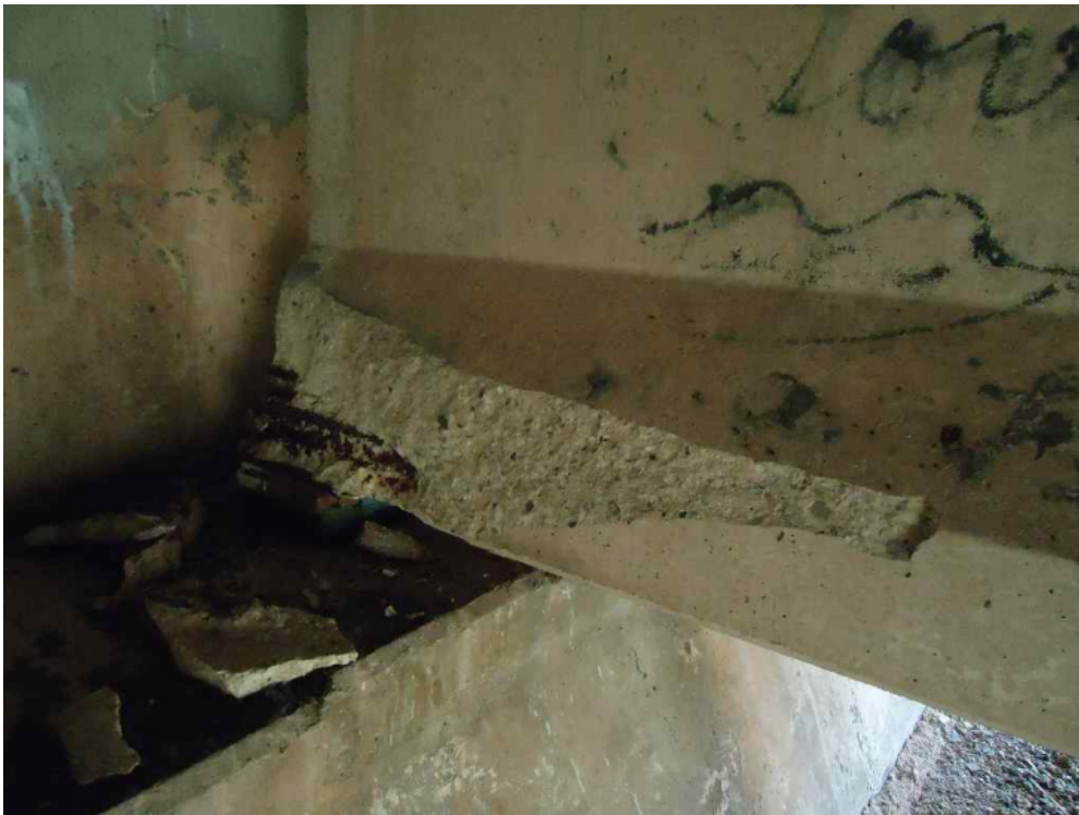
Spalling in Girder 2 at South abutment
