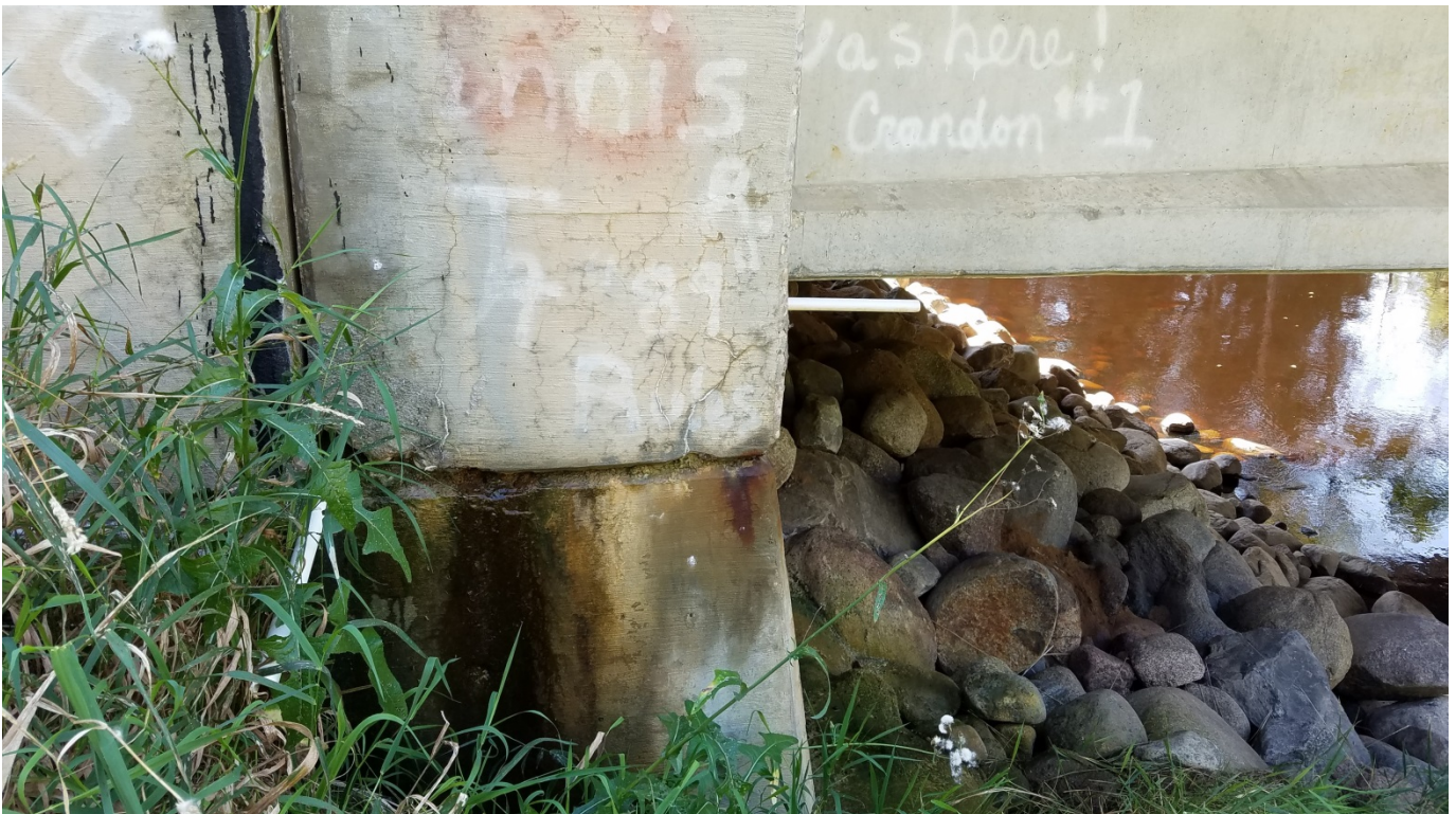
Figure 12 – Drain pipes in East Abutment
