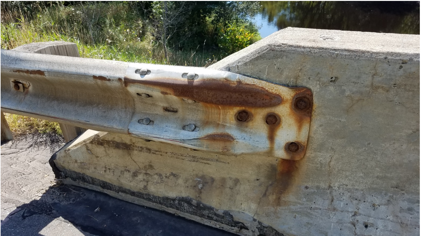
Figure 16 – Thrie Beam Connection (Typical)
