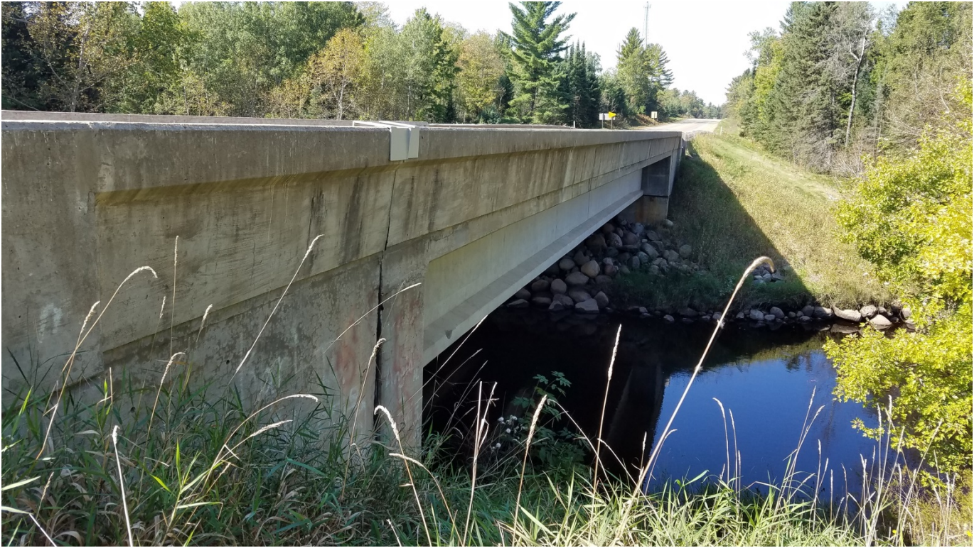
Figure 7- NE Wing Tipping
