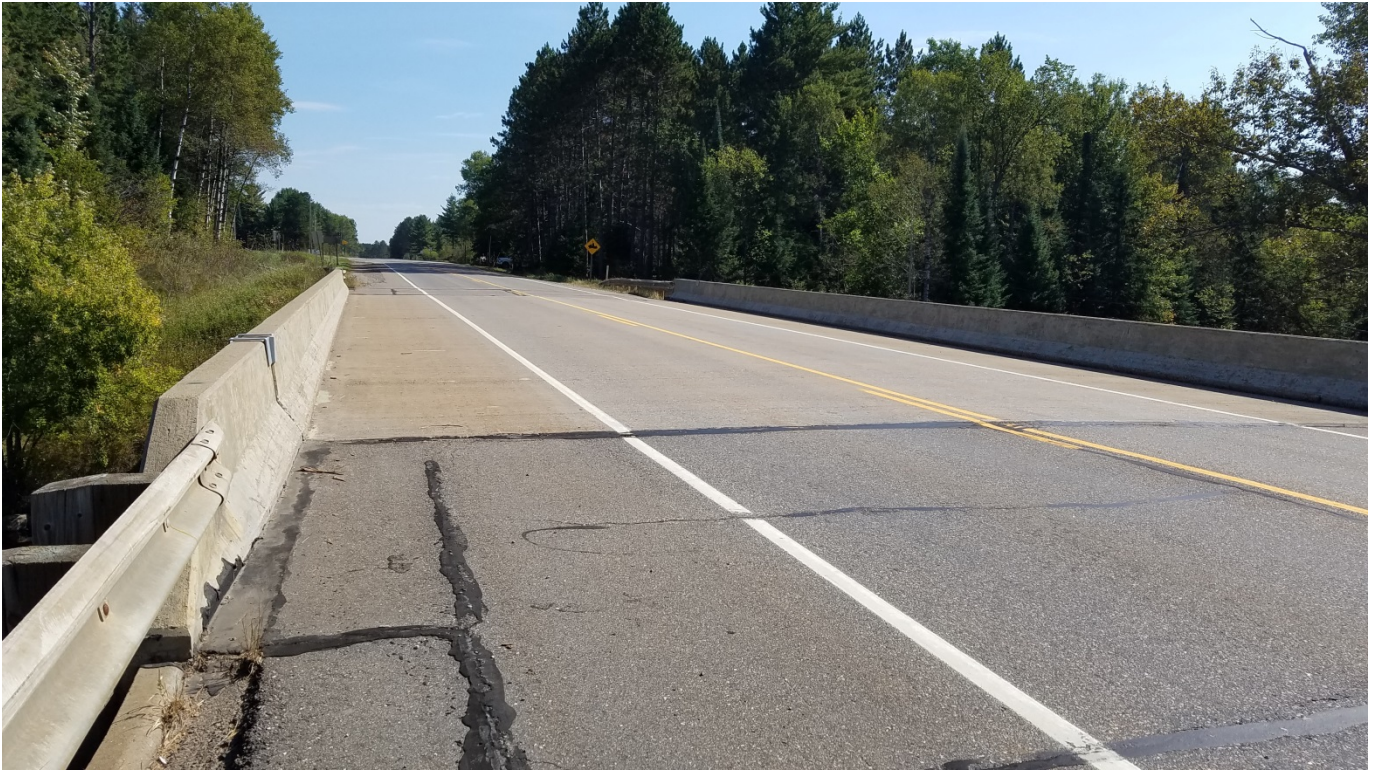
Figure 9- SW Wing Tipping
