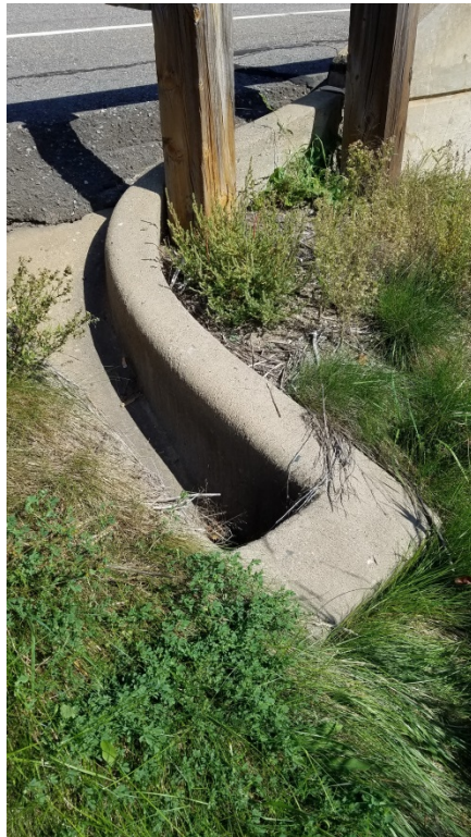
Figure 20 – Surface Drain at Southwest Corner
