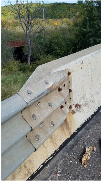
Figure 12 – Thrie Beam Connection (Typical)
