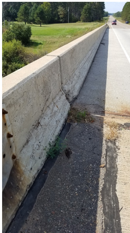
Figure 10 – Concrete Parapet (Typical)
