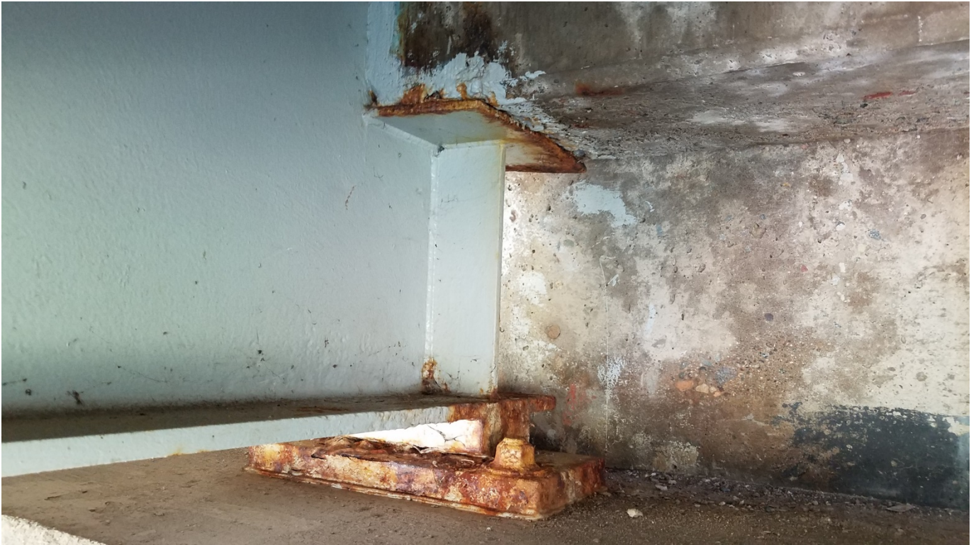
Figure 14 – Bearing (Typical)
