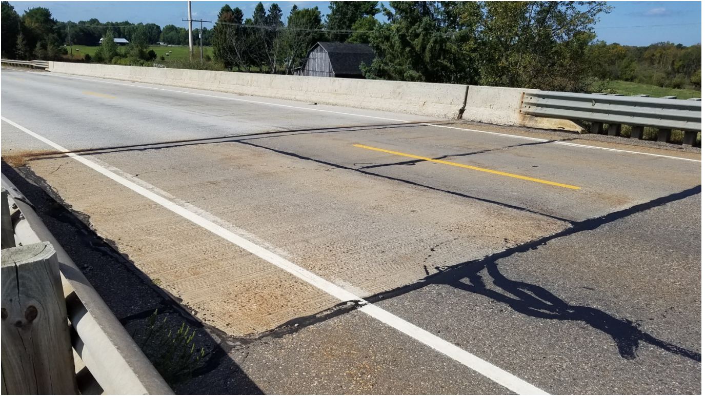
Figure 9 – Approach Slab Condition at East Abutment
