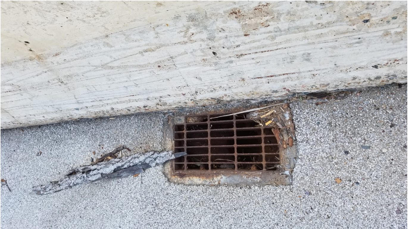
Figure 11 – Deck Drain (Typical)
