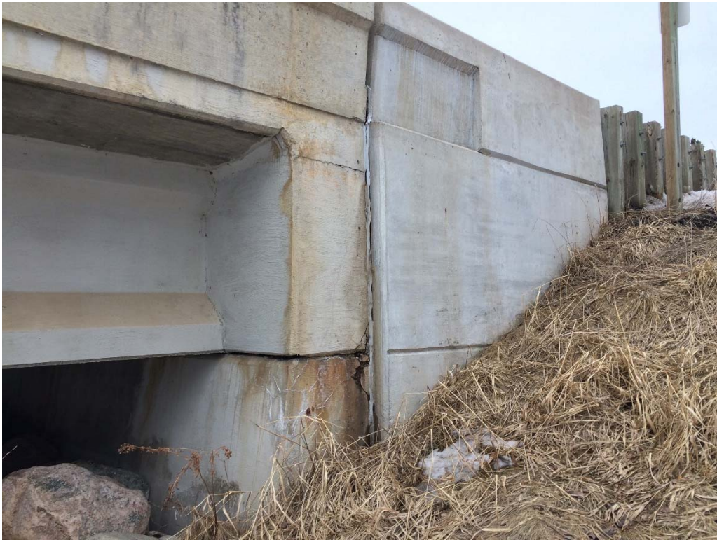
Surface repair on abutment, B-19-5
