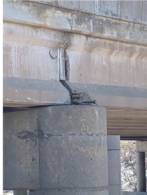
PIER 1 GIRDER SPALL
