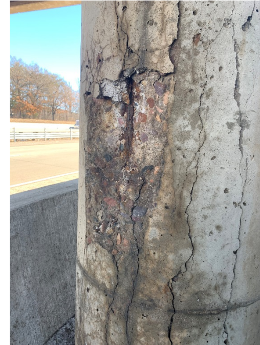
PIER 1 DETERIORATION
