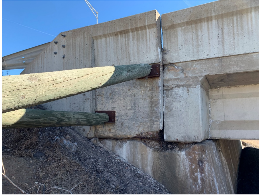
NW WING TIMBER SUPPORTS
