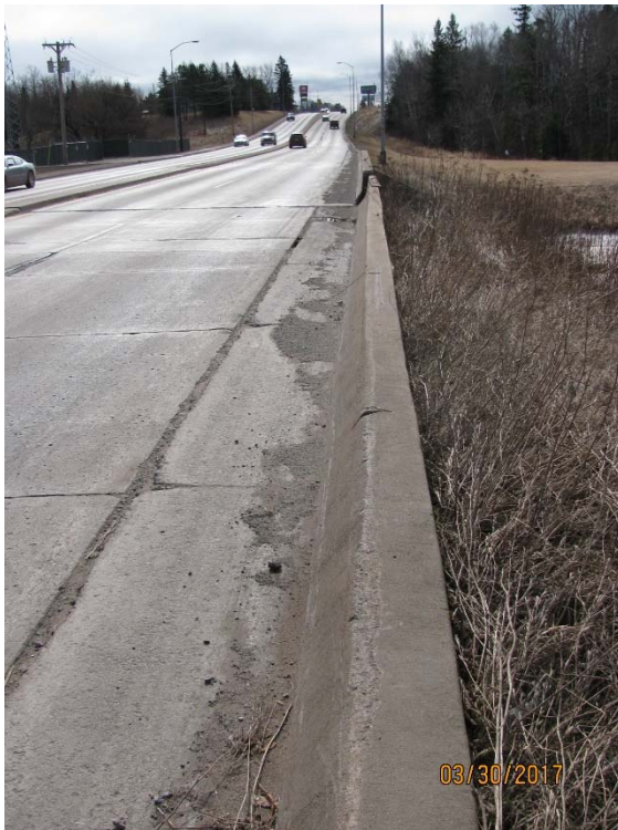
Photo 7 Parapet West Side Looking South
