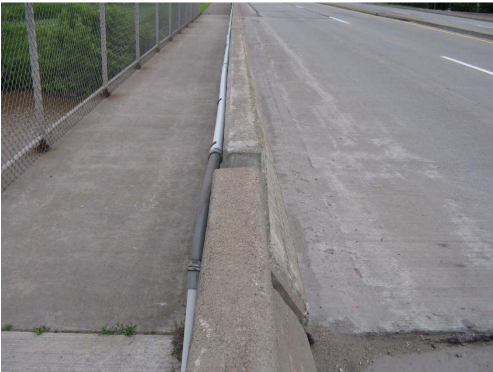
Photo 4 Parapet NE Quad
