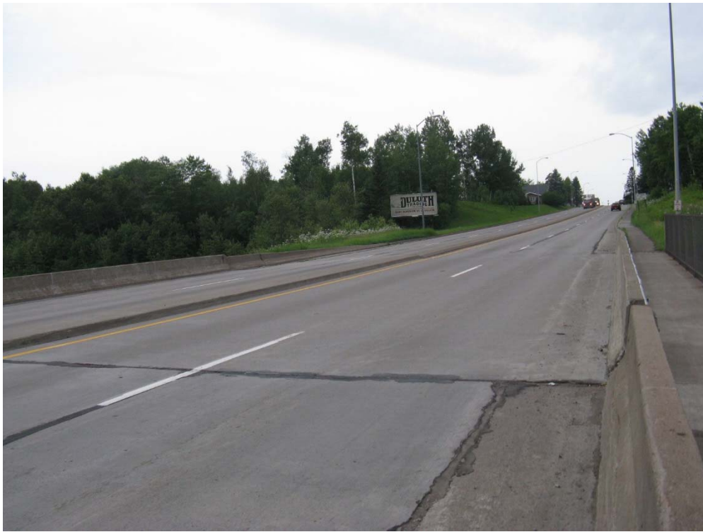
Photo 1 Parapet East Side Looking North
