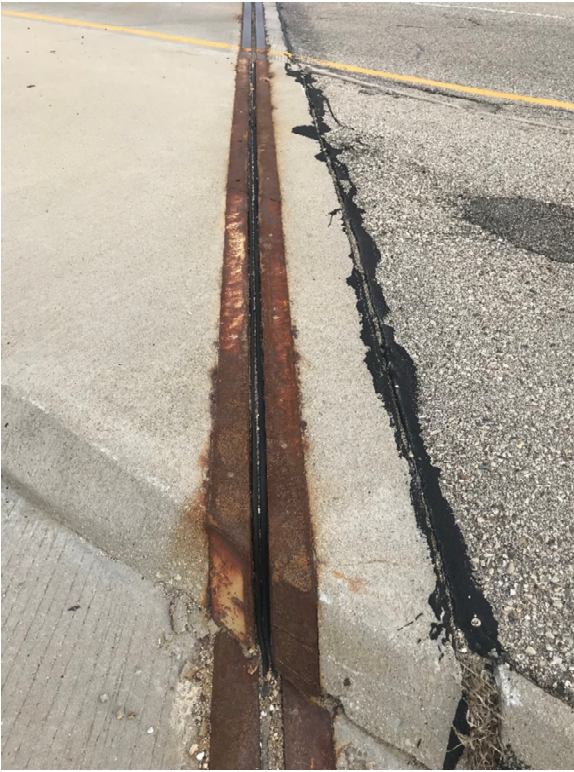
Photo 5. Expansion Joint – E. Abut. Median
