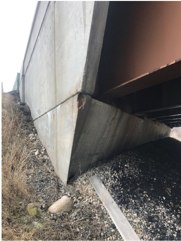
Photo 21. Corner Spall at E. Abutment Wing 3 (NE Corner)
