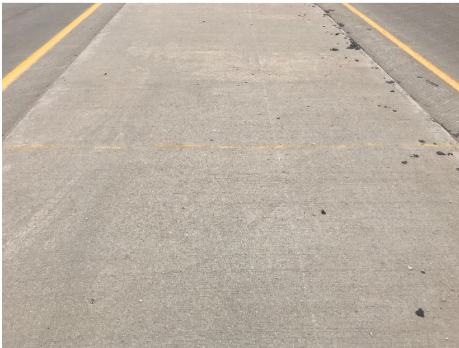
Photo 11. Typical Epoxy Sealed Cracks in Median
