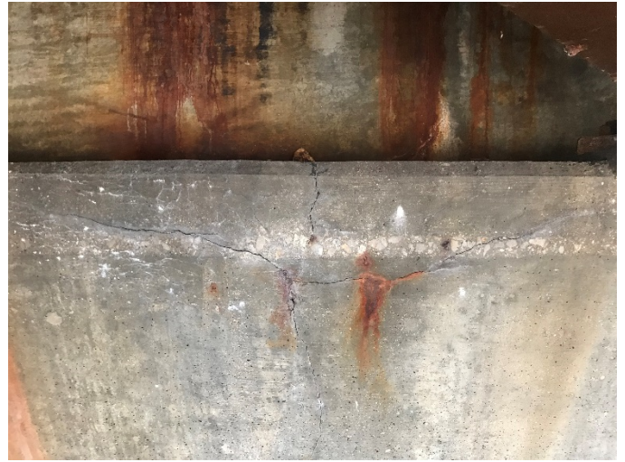
Photo 18. Typical Delamination at W. Abutment
