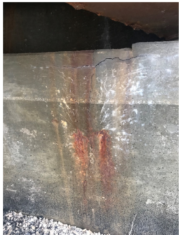
Photo 24. Typical Delamination at E. Abutment
