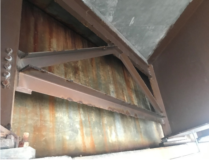
Photo 17. Diaphragms and Staining from Joint Leakage
