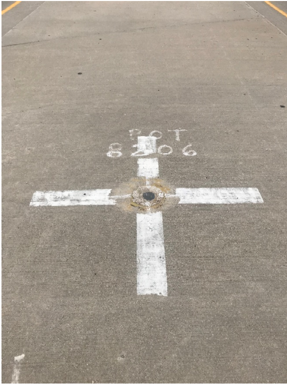
Photo 13. BM Cap in Median, Near CL Pier
