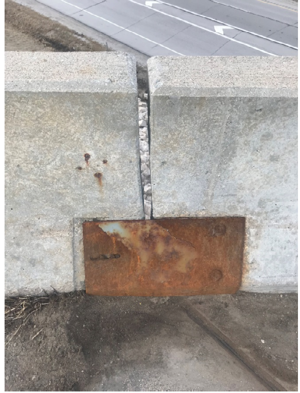
Photo 6. Typical Parapet Cover Plate
