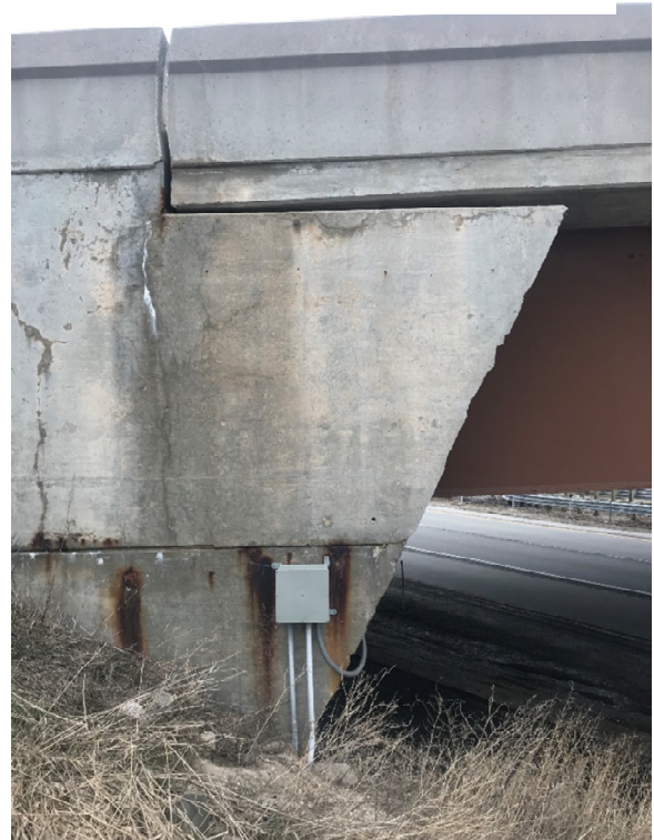
Photo 16. Access Box and Conduit at Wing 1, Assumed to Attach to Weather Station
