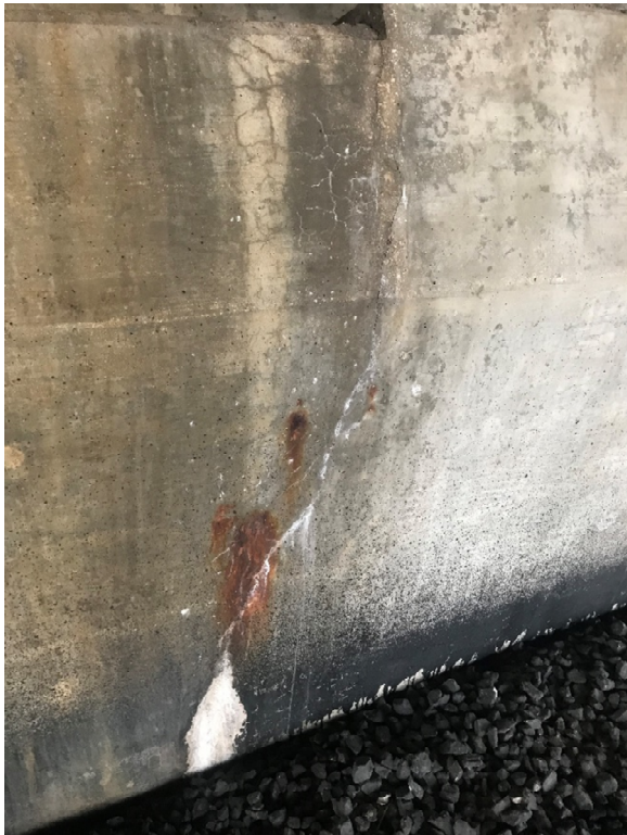
Photo 19. Typical Vertical Cracks in W. Abutment
