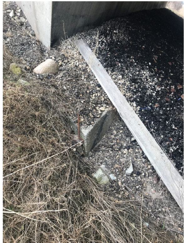
Photo 22. Exposed Footing at E. Abutment Wing 3 (NE Corner)
