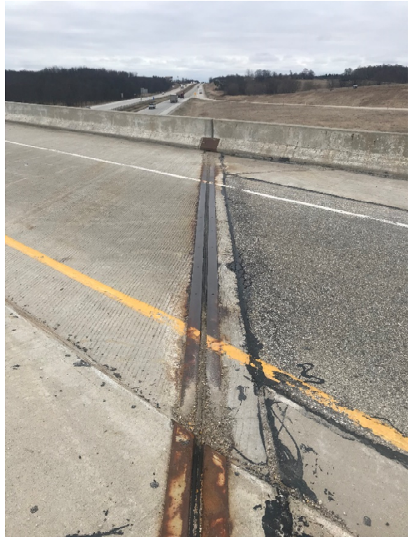
Photo 8. Expansion Joint – W. Abut. Eastbound
