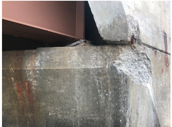
Photo 20. Corner Spall at E. Abutment Wing 4 (SE Corner)
