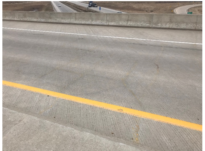
Photo 12. Typical Epoxy Sealed Cracks in Deck
