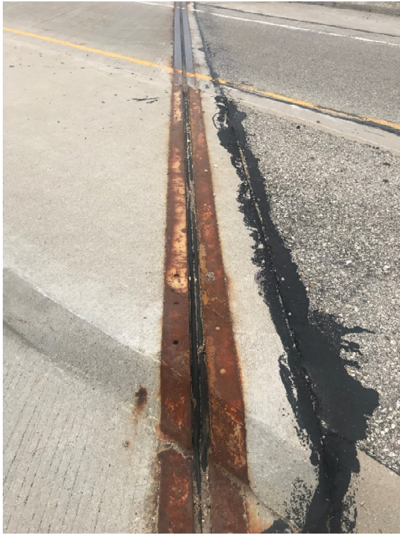
Photo 9. Expansion Joint – W. Abut. Median
