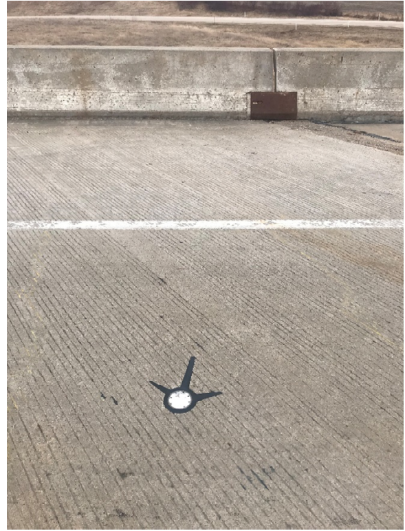
Photo 14. Cap in Deck, Assumed to Connect to Conduit Attached to W. Abutment
