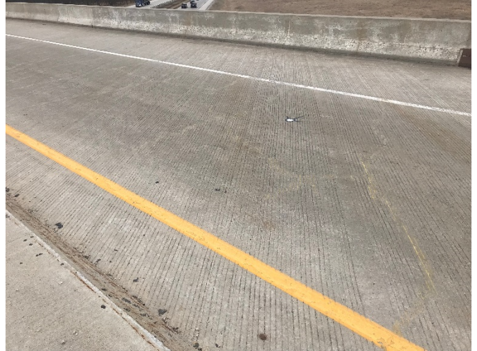
Photo 10. Typical Epoxy Sealed Cracks in Deck
