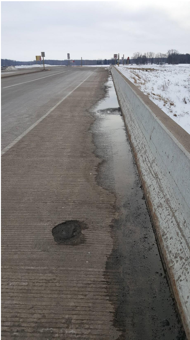
West end of deck looking south - spalling
