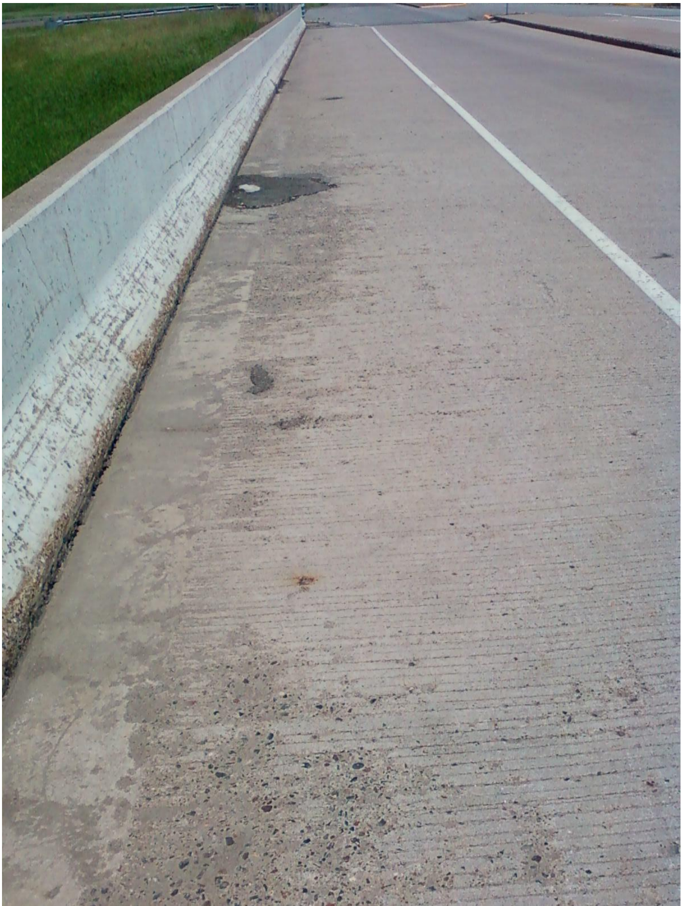
NW end of deck – Asphalt patch
