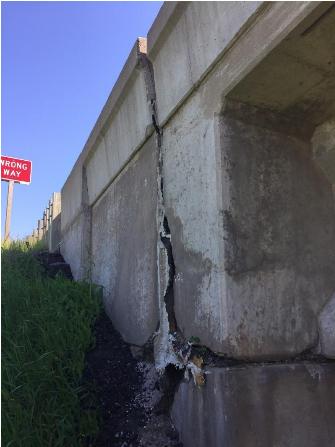
NW Wing – Tipping and Spalling
