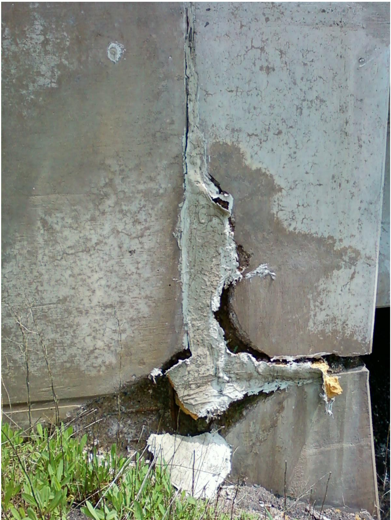
NW Wing – Spalling
