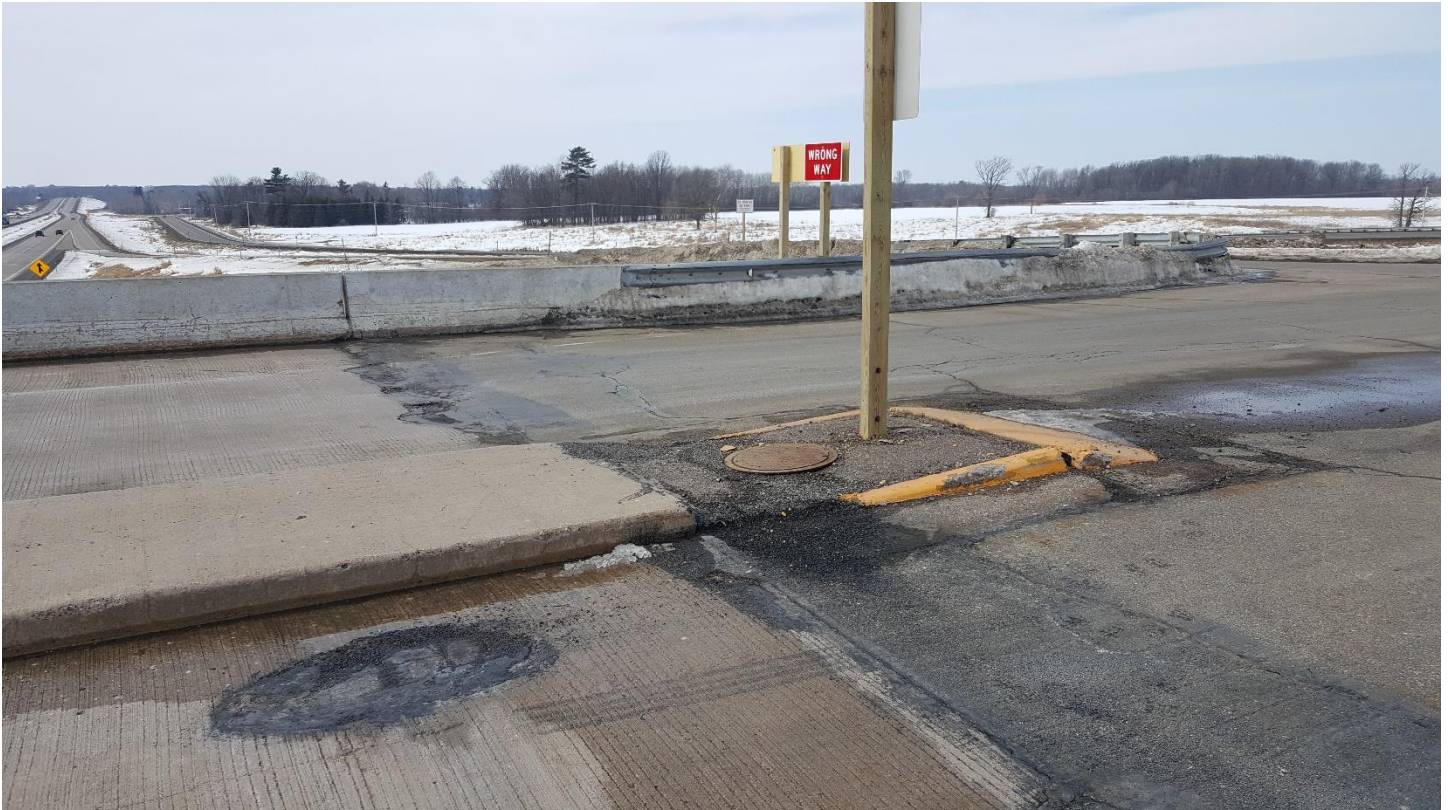
North End of Deck – Asphalt patch
