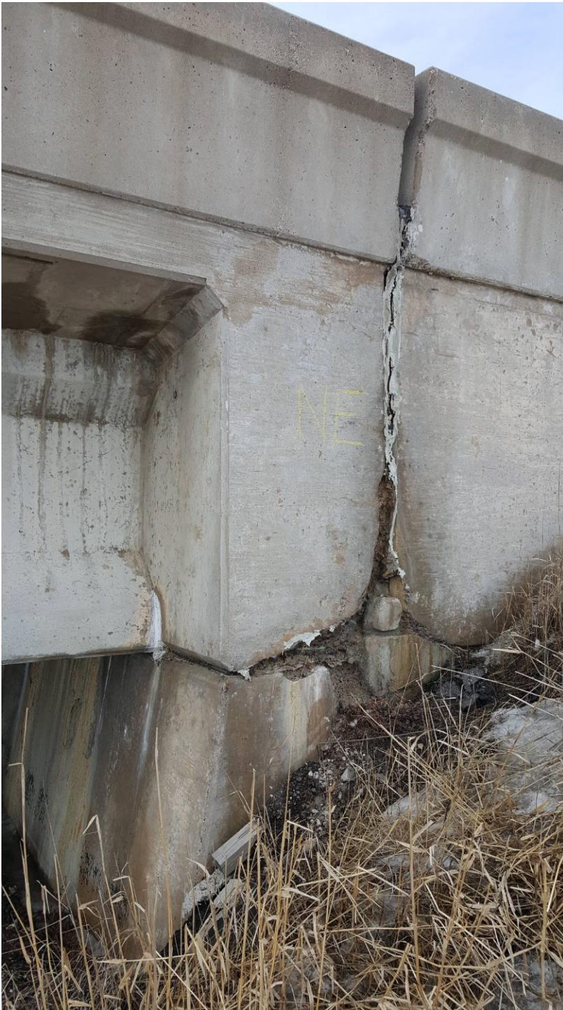
NE Wing – Tipping and Spalling
