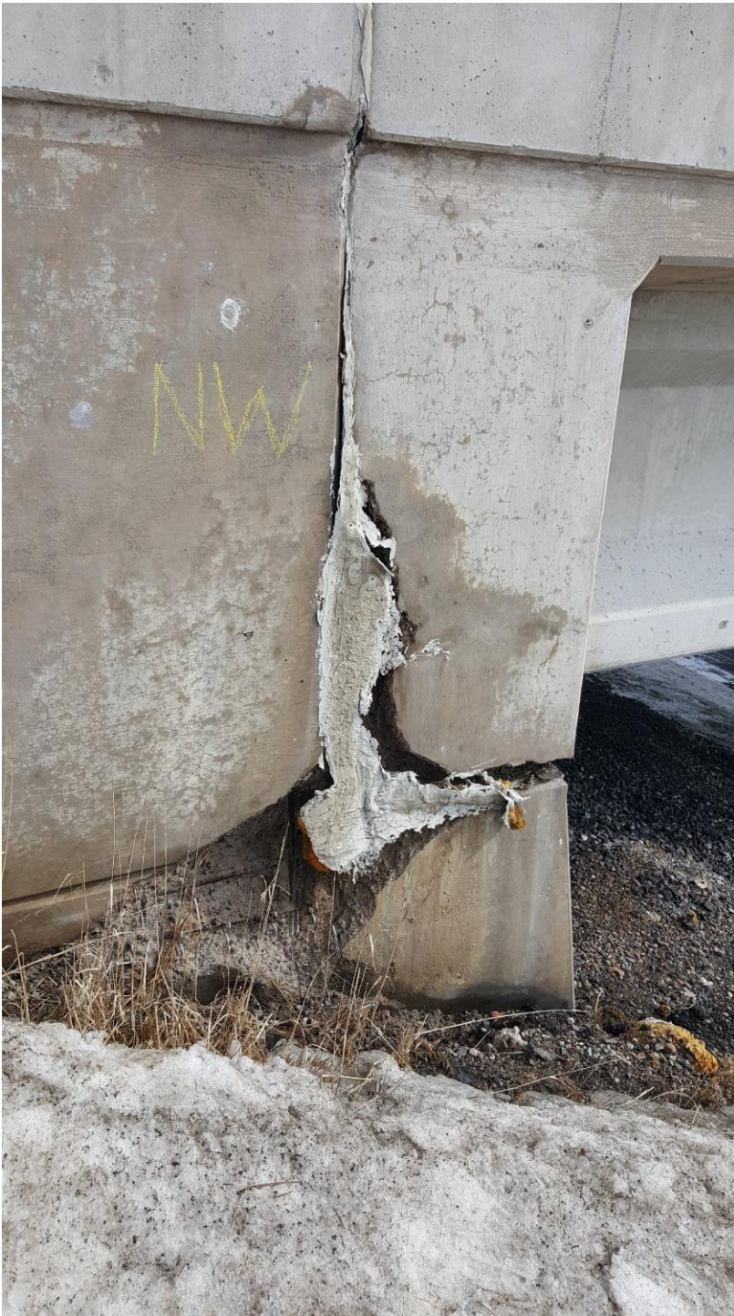
NW Wing - Spalling
