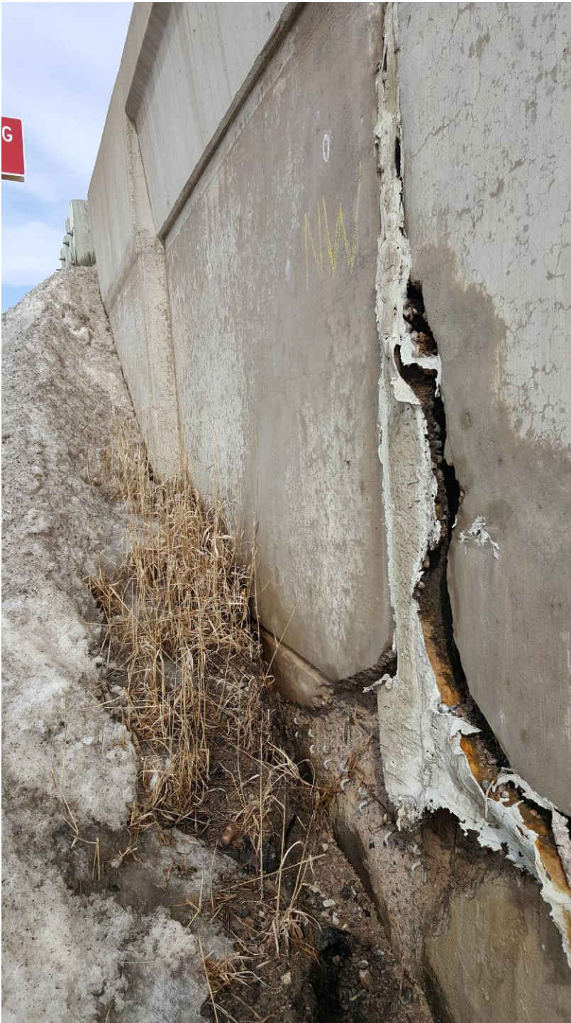
NW Wing – Spalling
