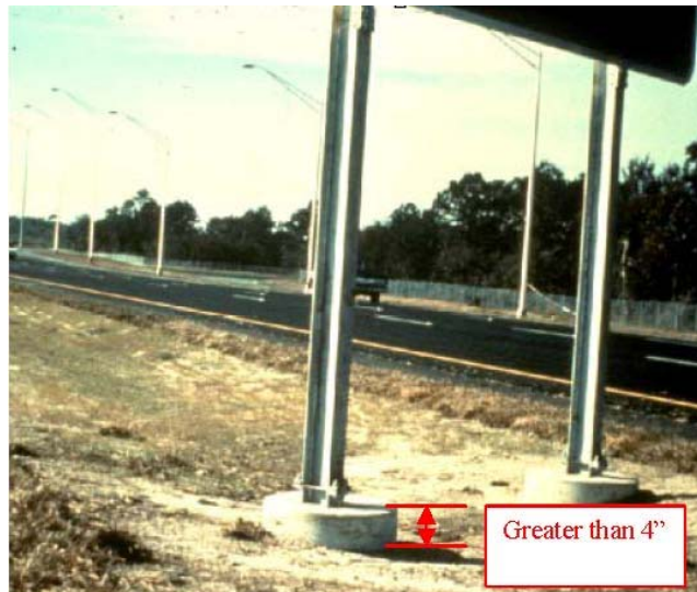
Figure 25.4 Improperly Installed Concrete Footing 3
