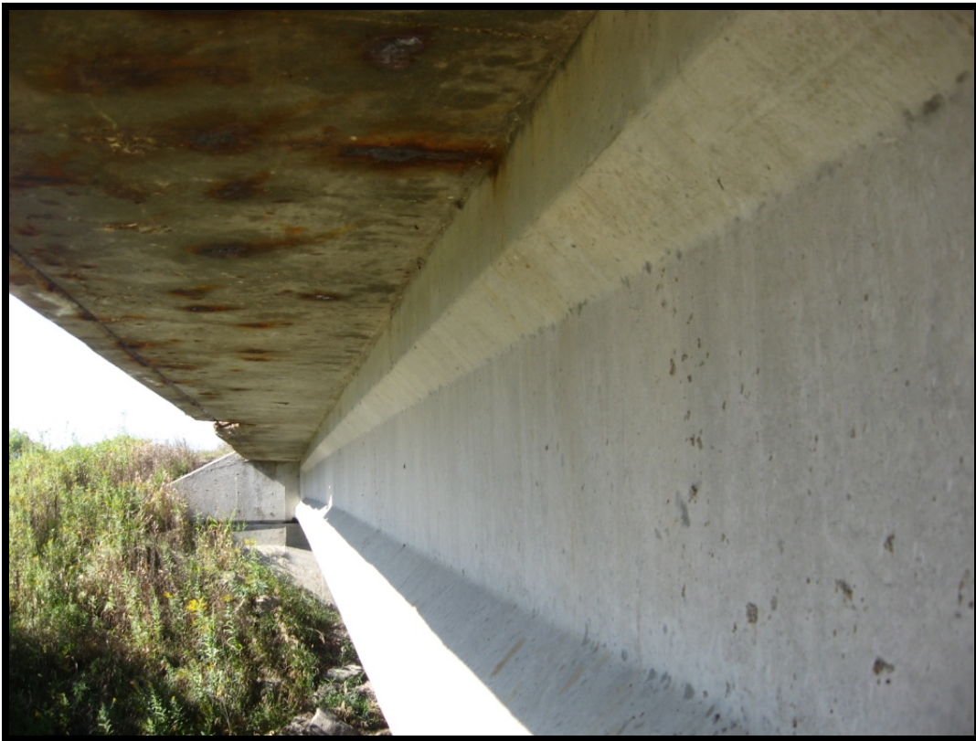
Figure 7-South abutment-bottom of bridge deck and concrete beam (NB lane, looking south)
