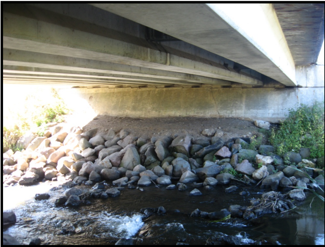
Figure 3-South abutment and concrete beams
