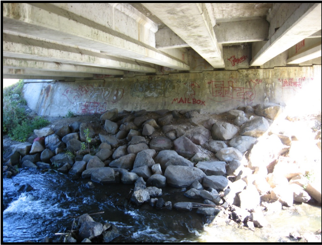
Figure 2- North abutment and concrete beams
