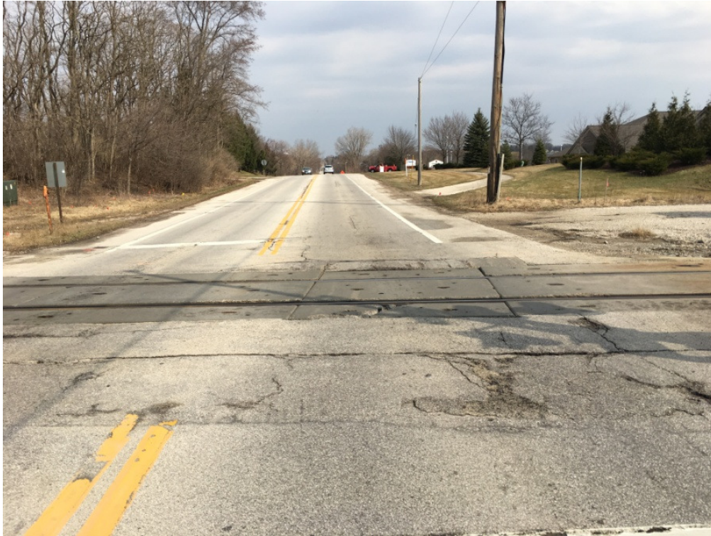
Photograph 7 Crossing Surface (Facing North)
