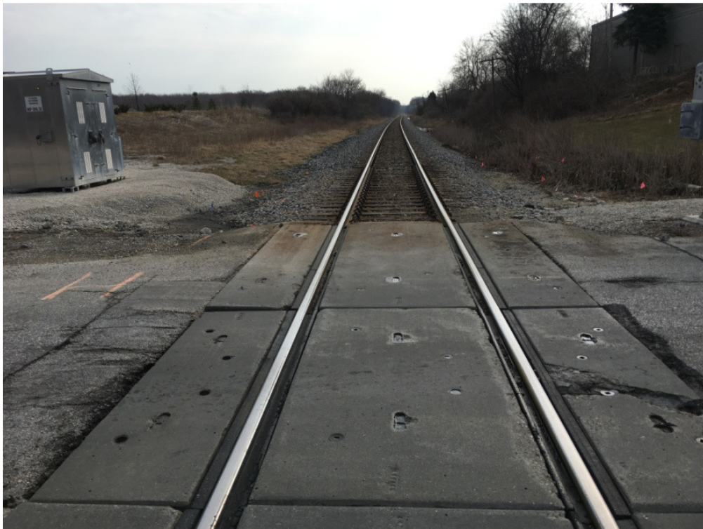
Photograph 6 Track (Facing East) Date: March 24, 2017
