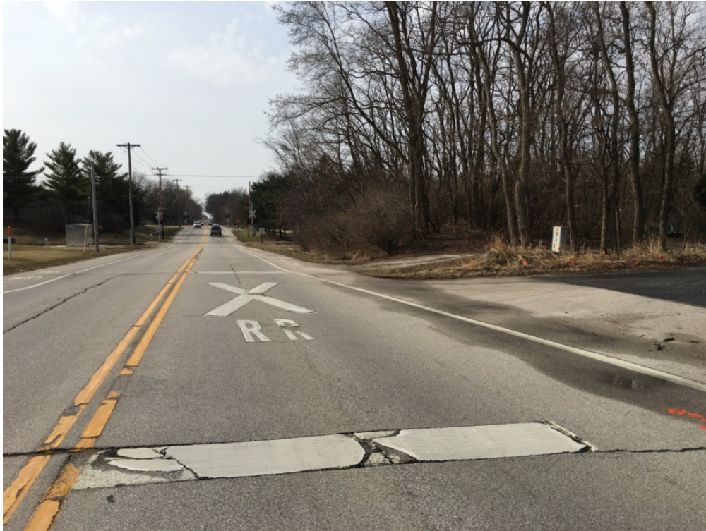
Photograph 15 Northwest Quadrant Crossing at Stopping Sight Distance (Facing Southwest) Date: March 24, 2017
