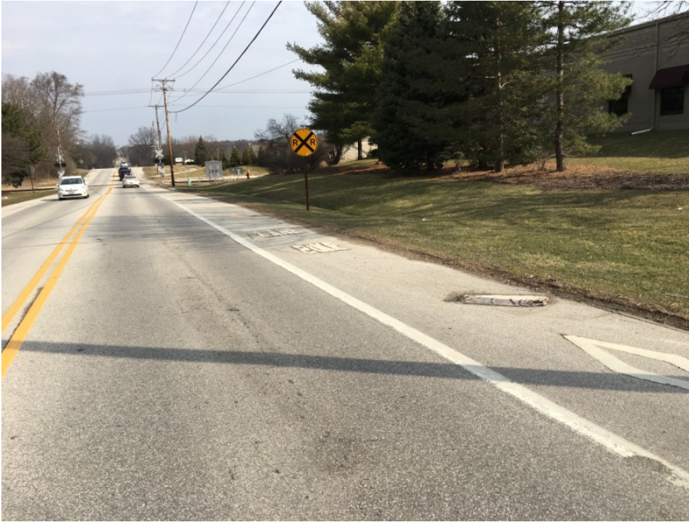
Photograph 3 Southeast Quadrant Crossing at Stopping Sight Distance (Facing Northeast) Date: March 24, 2017
