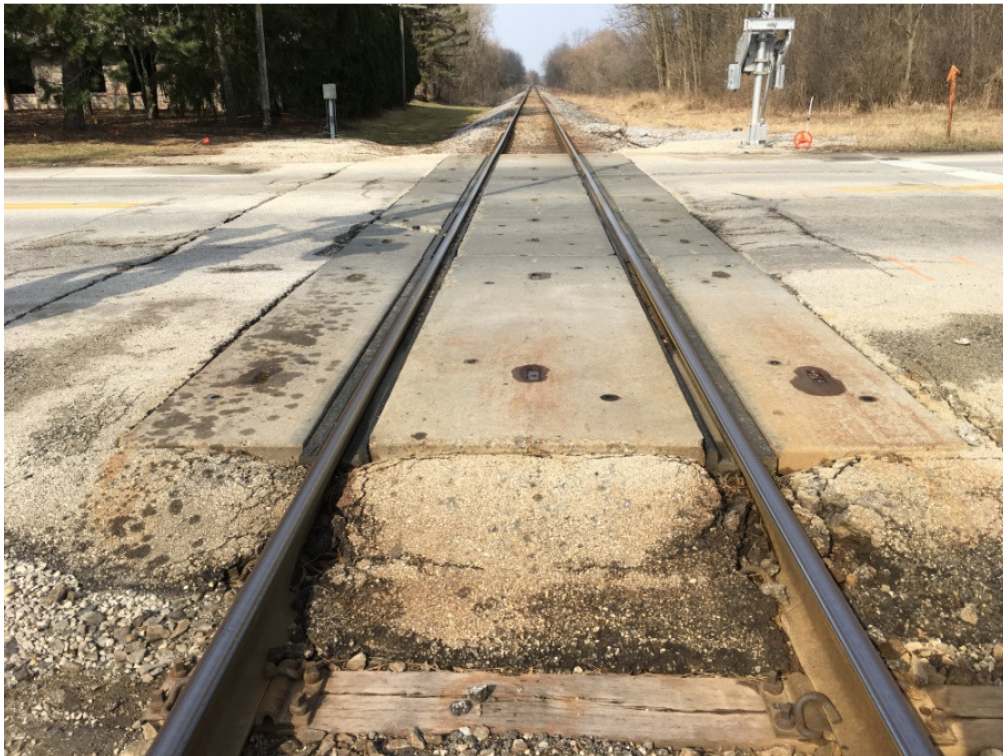
Photograph 8 Track (Facing West)
