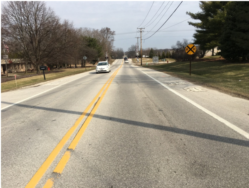
Photograph 18 Crossing at Stopping Sight Distance at 281 feet from crossing (Facing North)
