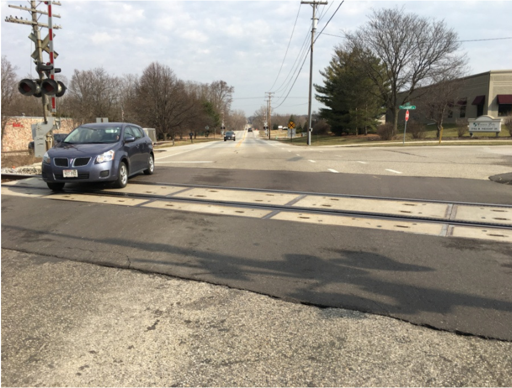
Photograph 1 Crossing beyond Stopping Sight Distance at 1,000 feet from crossing (Facing North) Date: March 24, 2017
