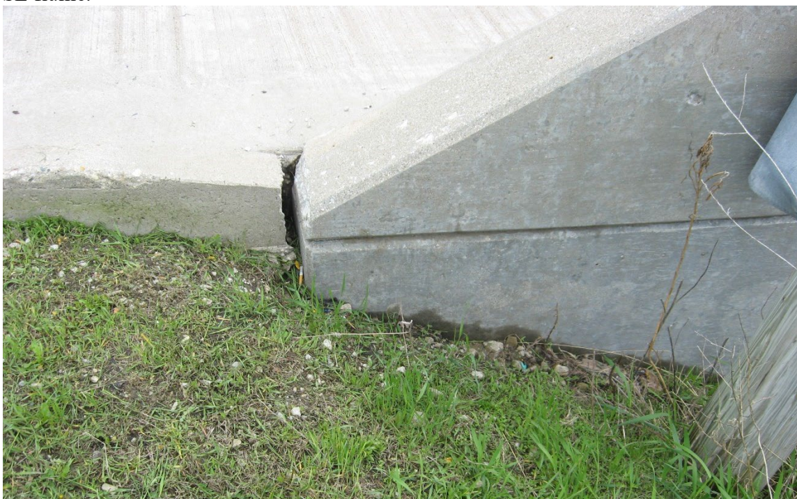
Joint at NE parapet and curb. Typical of all four corners.
