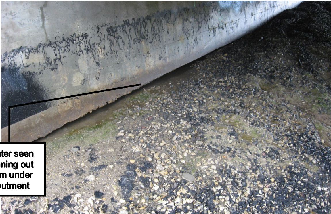
Settled slope paving at east abutment.
