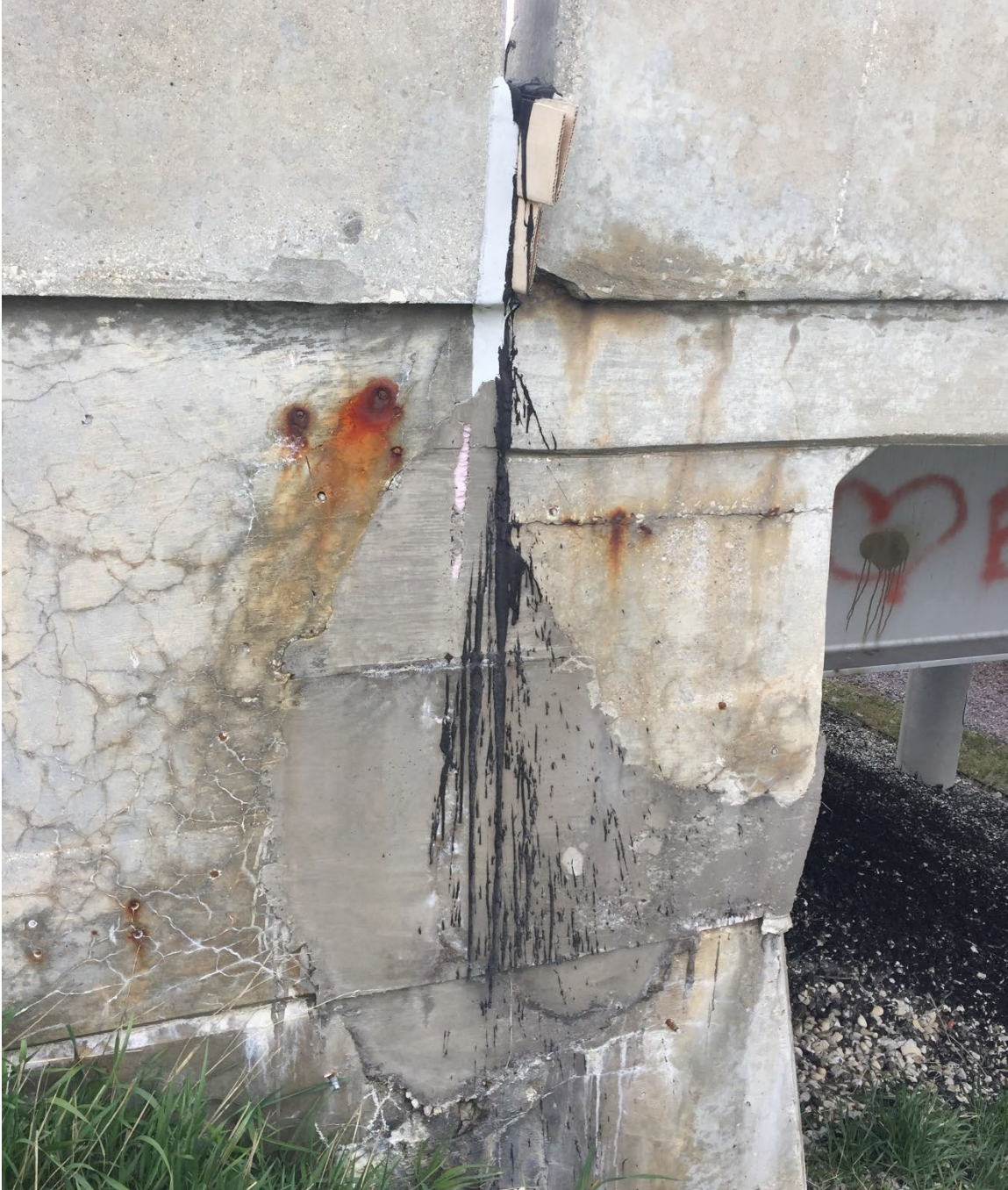
Concrete patch on SW abutment corner.
