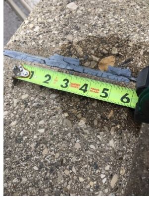
Gray caulk in parapet expansion joint, sidewalk joint
