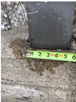
Gasket under railing attachments
