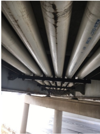
Utilities encased in PVC piping
