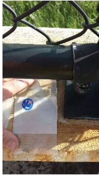
Caulk around fence attachment plates
