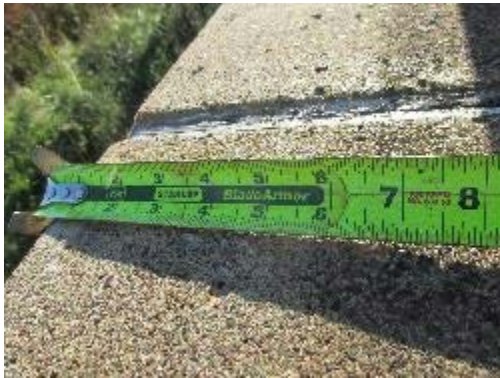
Caulk in parapet expansion joint
