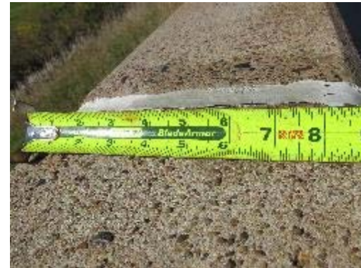
Caulk in parapet expansion joint
