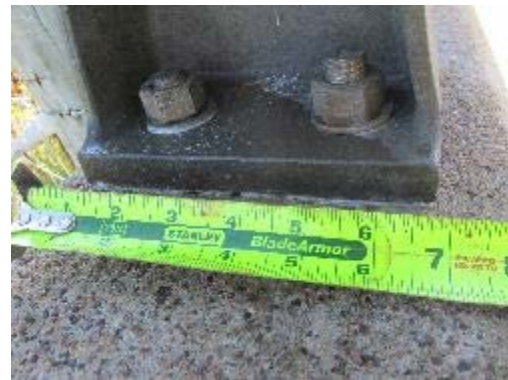
Gasket under railing attachment plate
