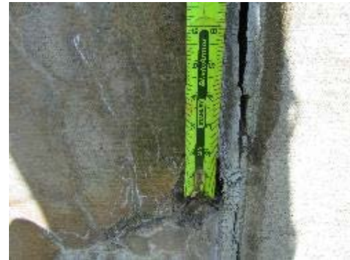
Caulk in abutment joint
