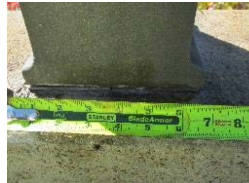
Gasket under railing attachment plate
