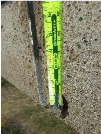
Caulk in parapet expansion joint
