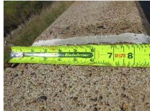
Caulk in parapet expansion joint
