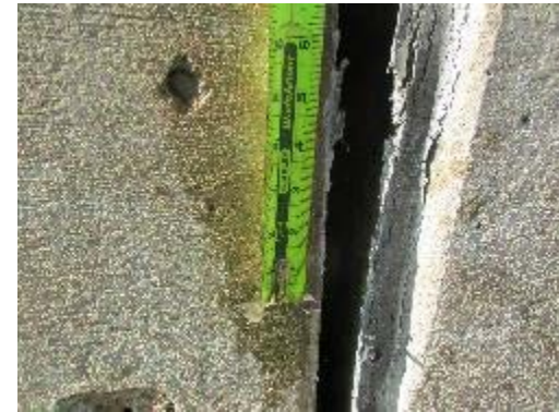
Caulk in abutment joint
