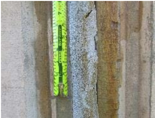
Caulk in abutment joint
