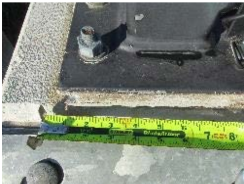
Caulk around fence attachment plate
