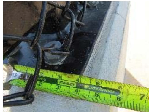
Caulk around bolts in attachment plate
